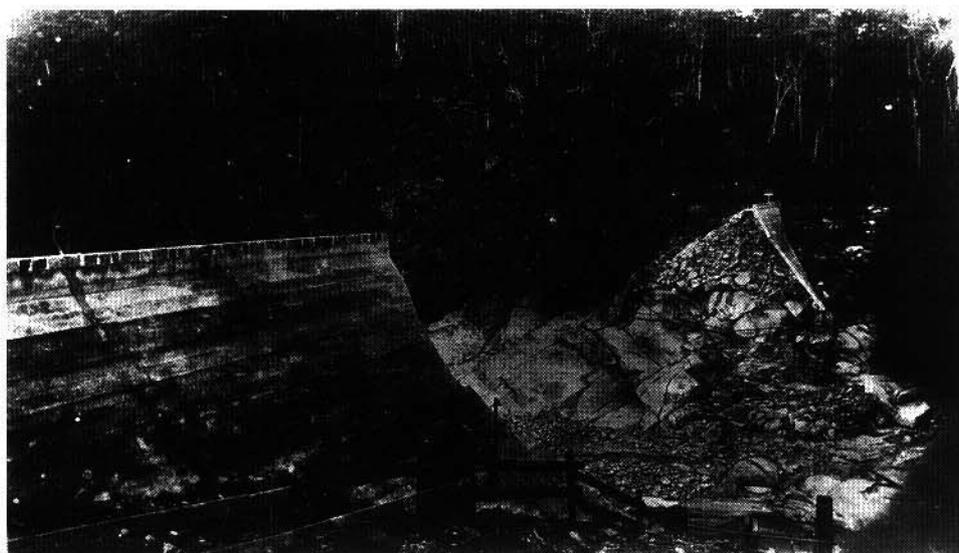
Briseis Dam was designed to have spill water flowing over and through the downstream rockfill but a flood of the rarity and size that occurred on April 4th 1929 was not envisaged by the designer. Briseis Dam failed due to prolonged overtopping by a flood much greater than the design flood. Water flowing over and through the rockfill carried away material critically weakening the dam and causing its ultimate rapid failure (Photo 1).
