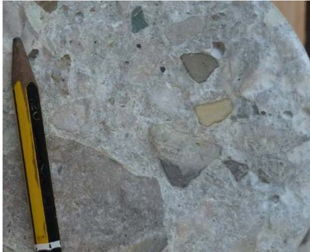
Fig. 4.18 - Dark rims surrounding reactive dolomite particles in a dam concrete core.
