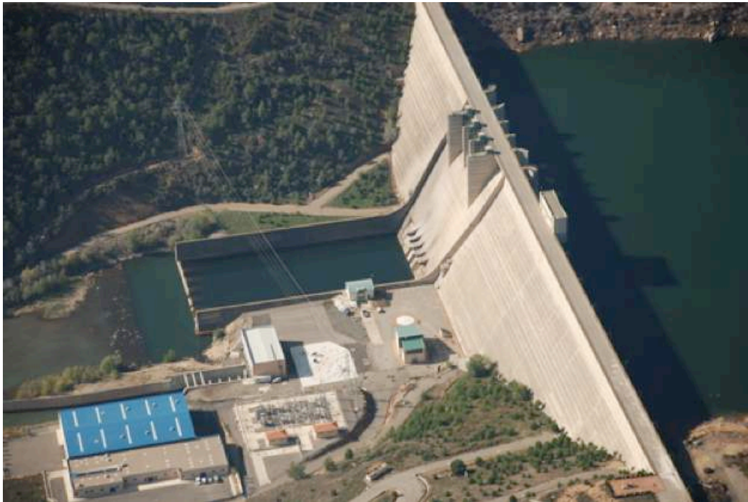
Figure 3-1 Gravity dam of RCC (Rialb, Spain: Height 99 m, Volume 1.02 Mm 3 )
