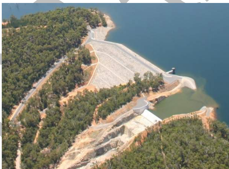
Figure 5-3: Embankment dam with spillway in adjacent valley
