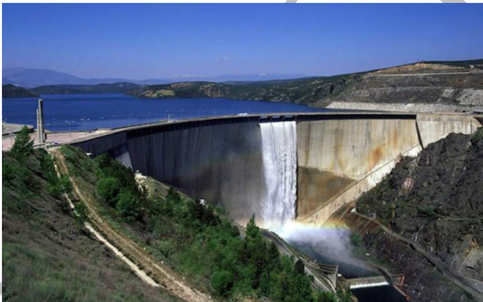
Figure 3-11 Double curvature arch dam in CVC (Atazar, Spain, 130 m high)
