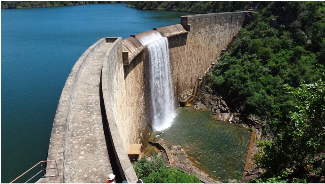
Figure 3-21 Rubble Masonry Concrete Arch dam, 42 m high (Lucilia Poort, Zimbabwe)
