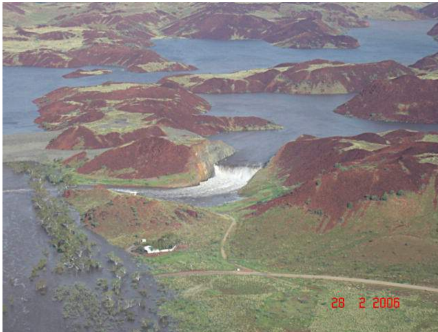
Figure 5-4 Harding Dam; unlined spillway was used as a source of rockfill
