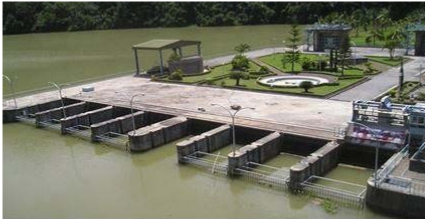
Fig. 3.62 Raking system in Bakaru intake
