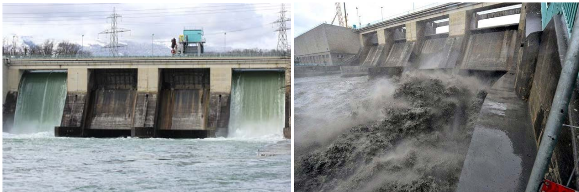
Fig. 3.40 Verbois spillways and outlet gates
