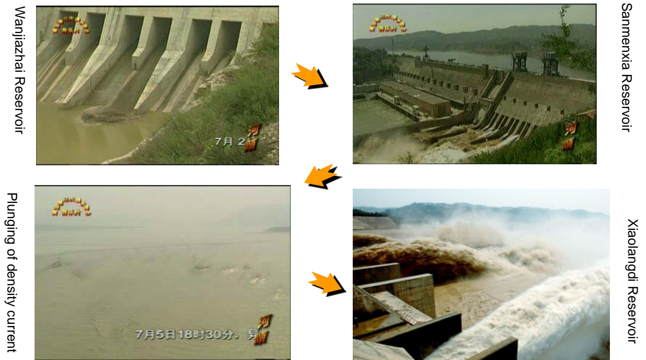
Fig. 3.32 Process of density current flow modeled by Wanjiashai, Sanmenxia and Xiaolangdi Reservoir
