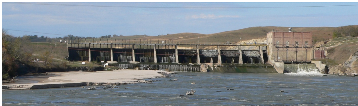
Fig. 3.125 Downstream face of Spencer Dam spillway and powerhouse (public domain photograph)
