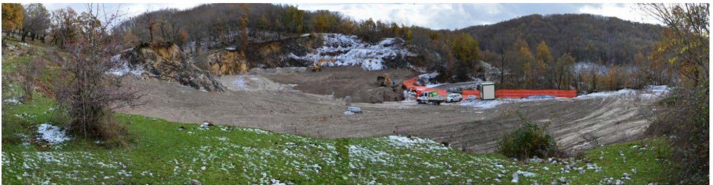
Fig. 3.78 During the removal of sediment
