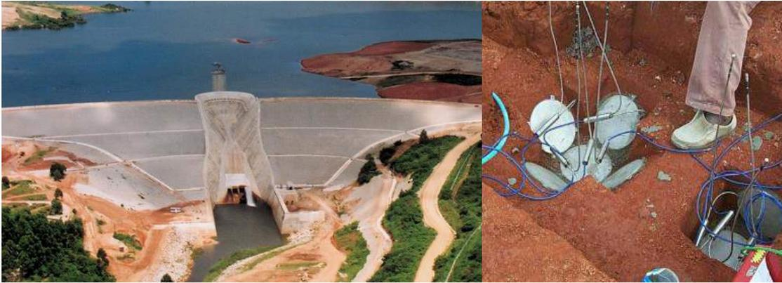
Fig. 1. Dam aerial view and layout of earth pressure cells
