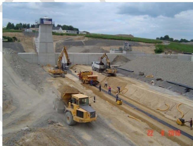
Figure 3.1 Earthwork sequence and following ACED placing (Rennersdorf Dam, Germany, 2010)
