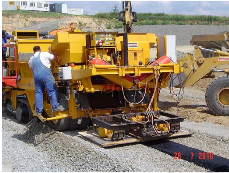
Figure 5.2 STRABAG Placing unit 3 rd generation with pre-compacting plates at paving works
