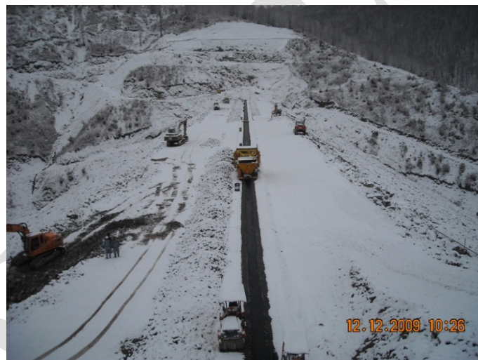
Figure 3.2 Knezovo dam, Macedonia, December 2009
