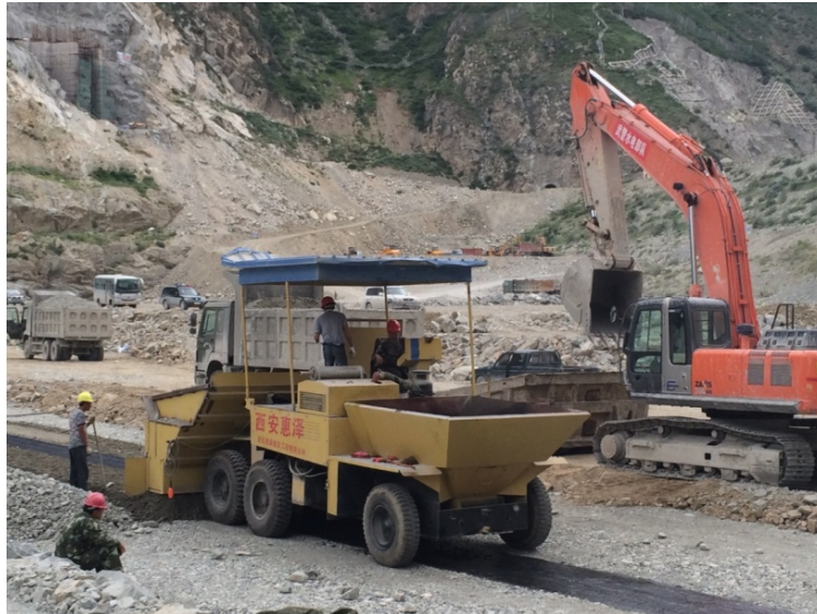
Figure 5.5 Xi'an Huize latest core paving machine in work, Huangjinping Dam, 2015
