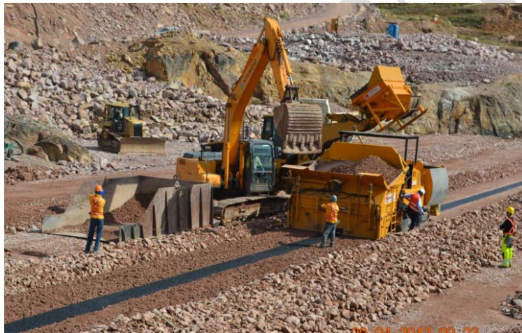
Figure 5.4 Veidekke core paving machine in work, Jirau Dam, Brazil, 2012
