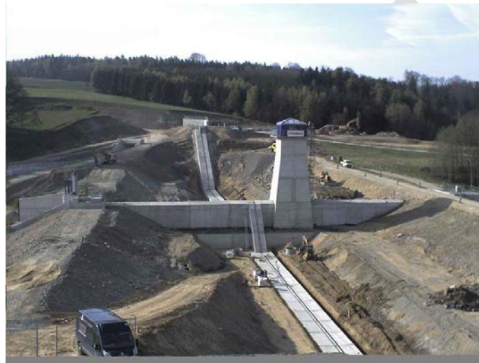
Figure 4.3 Concrete plinth construction (Rennersdorf Dam, Germany, 2010)
