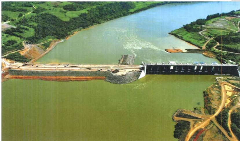
Figure B.7.3 Overview of dam and spillway
