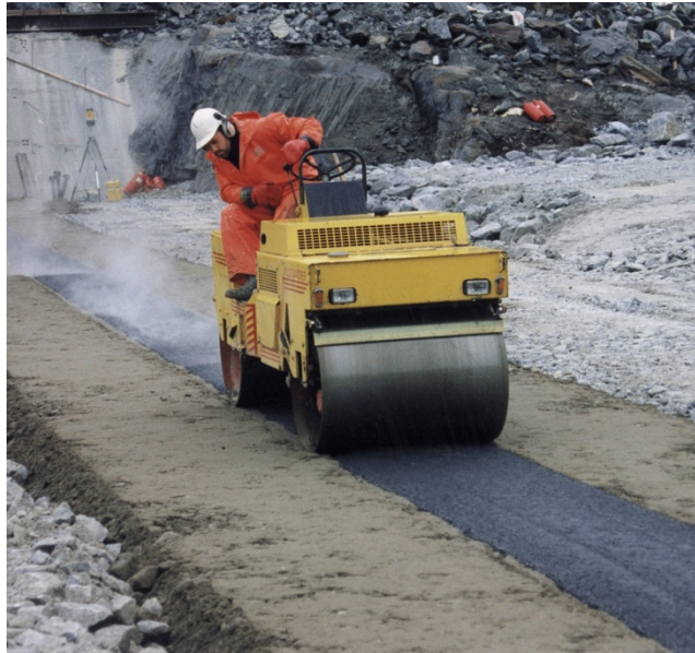
Figure 5.8 Final compaction of the asphalt concrete core
