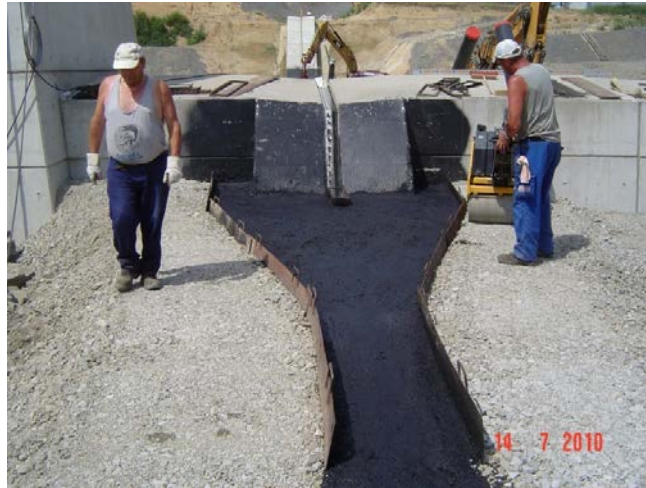
Figure 5.13 Manual placement and core widening adjacent to the abutments
