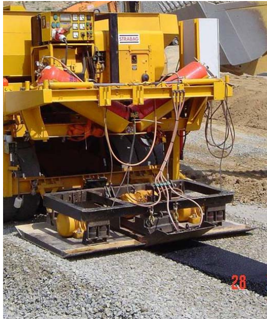
Figure 5.14 STRABAG Pre-compaction with vibratory plates
