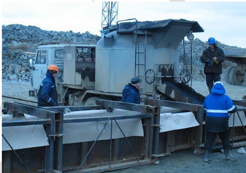
Figure C.2 Unloading of asphalt concrete mix from asphalt-truck into formwork
