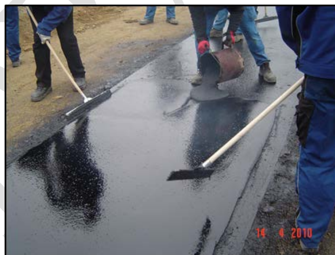
Figure 5.12 Mastic application on concrete plinth
