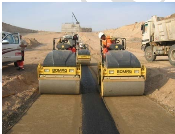
Figure 5.7 Compaction work at Murwani Saddle Dam, Saudi Arabia 2007
