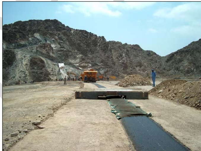
Figure 5.20 Temporary bridge for crossing the asphalt concrete core when required
