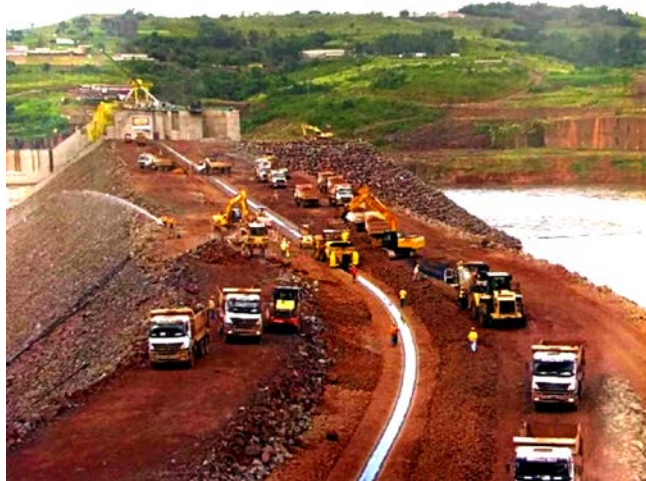
B.7.2 Work in progress
