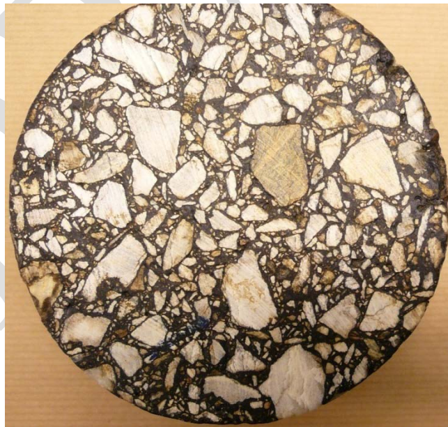
Figure 4.10 Drilled and cut core sample with floating coarse aggregates
