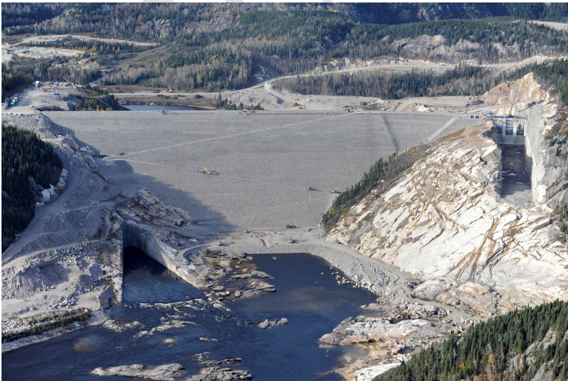
Figure B.8.4 Romaine-2 Dam Downstream Shoulder, Diversion Portal and Spillway
