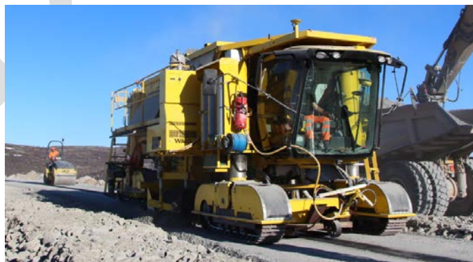
Figure 5.6 WALO's latest core paving machine in work
