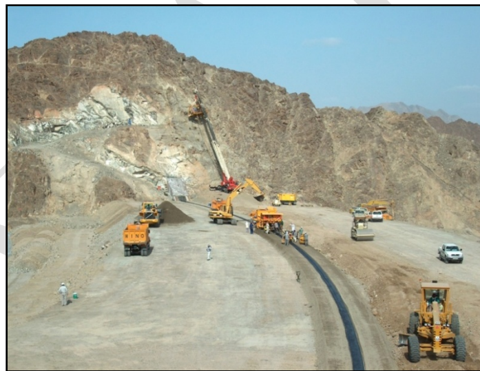
Figure 5.10 Hatta Dam, UAE, under construction, 2003
