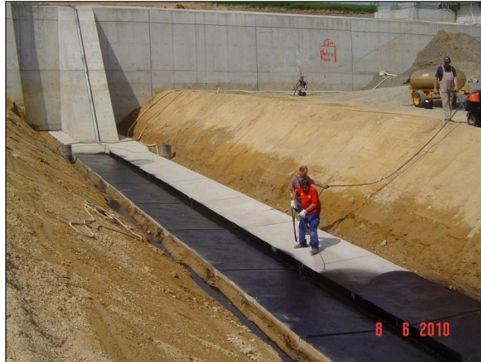
Figure 5.11 Tack coat spraying on concrete plinth prior to mastic application
