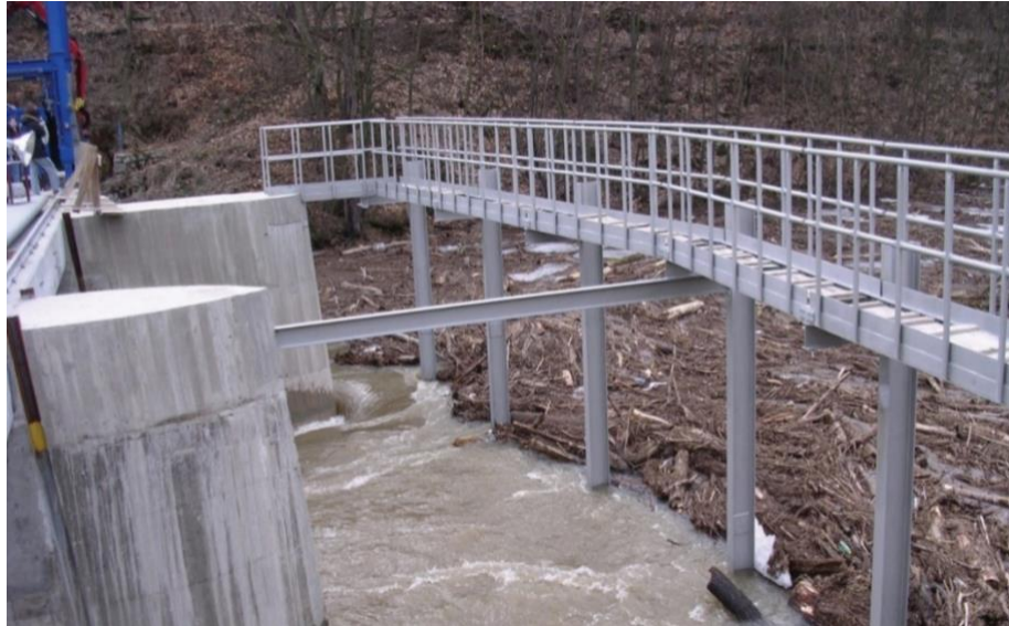
Fig. 4.15 Steel 'wood' rack frame at the Znojmo Dam in Moravia
