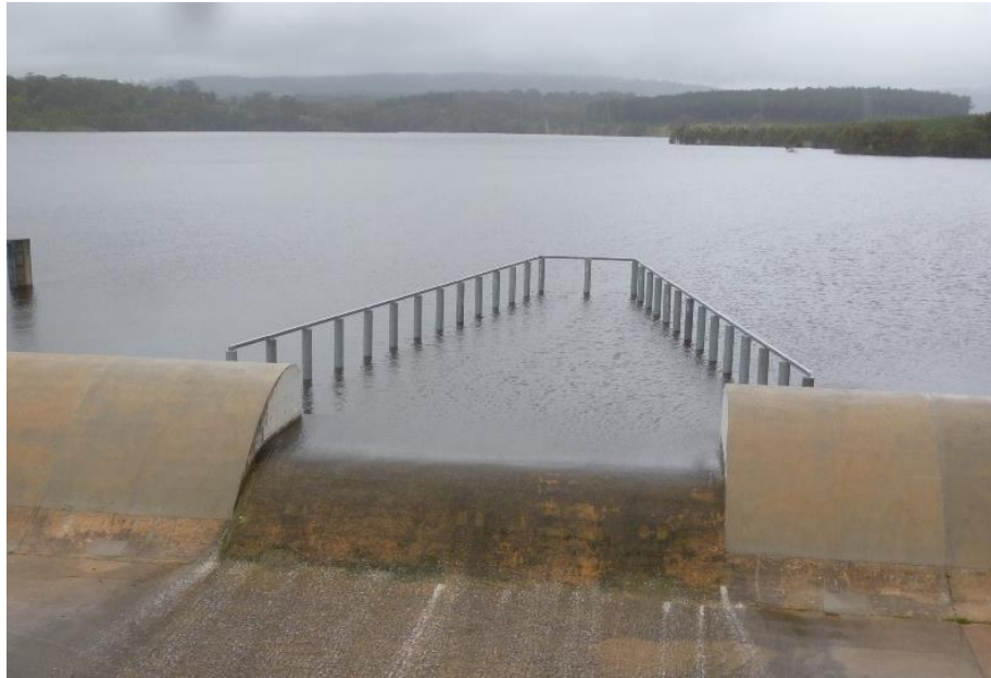
Fig. 4.11 A log collection structure on South Para Dam in South Australia
