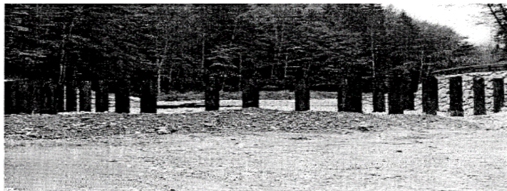
Fig. 4.5 "Treibholzfang" device on River Lainback (viewed downstream)
