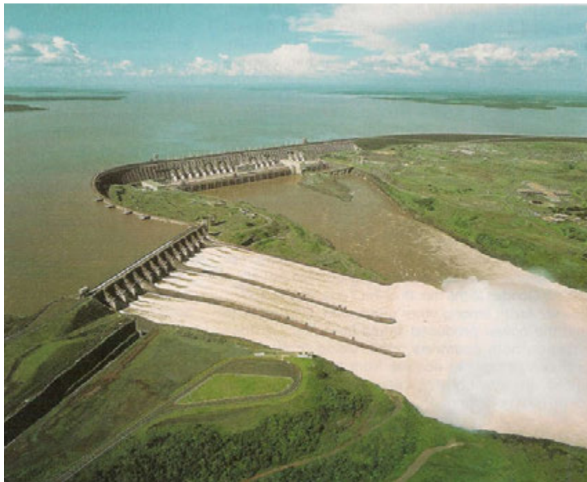
Fig. 2.1 – Itaipu Project (Brazil-Paraguay border) and its 62 200 m 3 /s spillway
