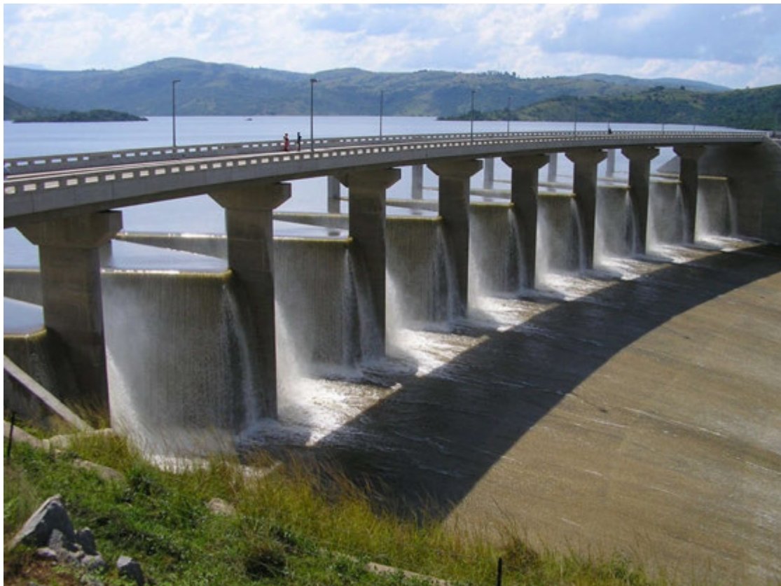
Figure 5.1 - View of the Labyrinth Spillway of Maguga Dam in Swaziland
