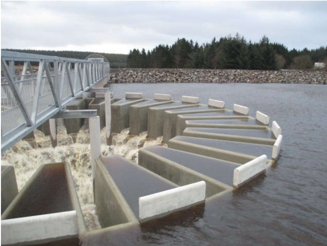
Fig 6.13 - Back Esk Reservoir spillway – PKW made of prefabricated concrete elements (Courtesy of Black and Veatch Ltd)
