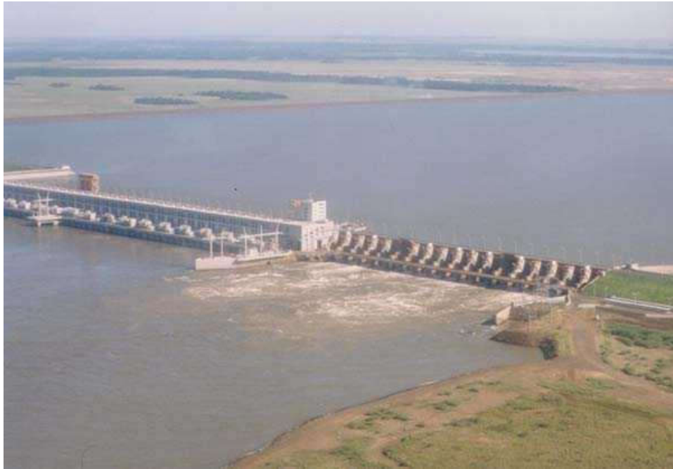
Fig. 2.7 - Yaciretá-Apipé Project – 816 m long powerhouse on the Paraná River next to the 55 000 m 3 /s main spillway - Argentina/Paraguay Border
