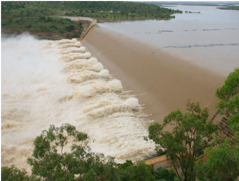
Fig. 2.5 – The 64 600 m 3 /s ungated spillway of the Burdekin Dam, Australia
