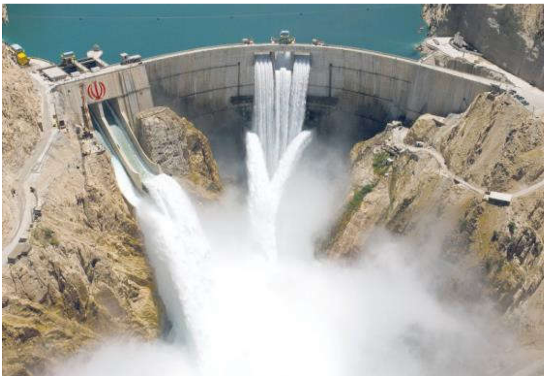
Fig. 10.1 - Karun III 205 m high concrete arch dam, service, auxiliary and emergency spillways (Iran)
