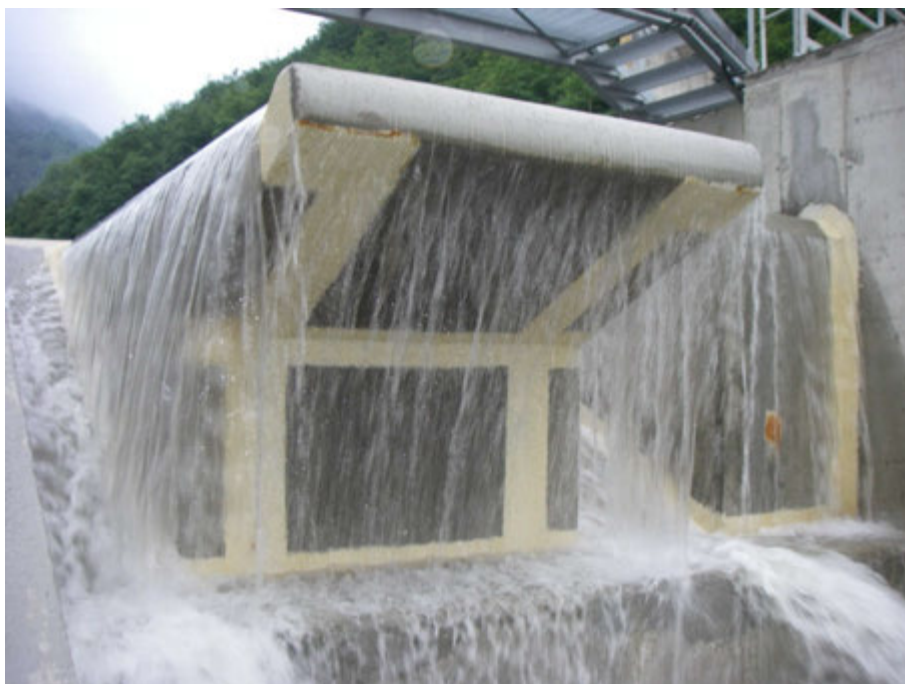
Figure 6.8 - Flow over the Escouloubre PKW (France) with an upstream head of a few cm (Photo courtesy of ULg-HECE)
