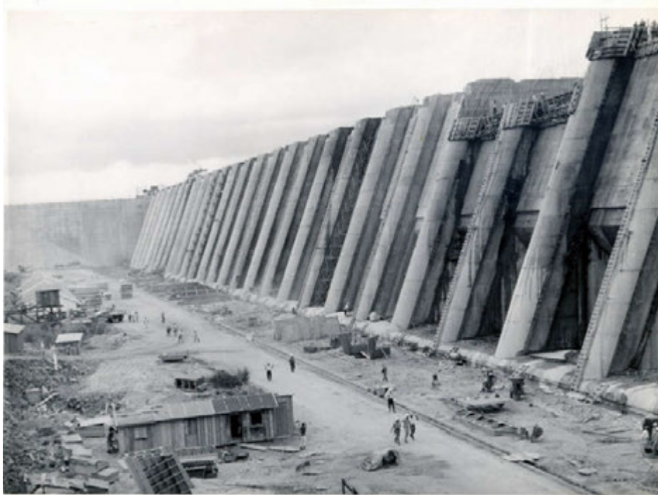
Fig. 2.10 - Jupirá Project – 44 000 m 3 /s bottom outlet spillway during construction (1967)
