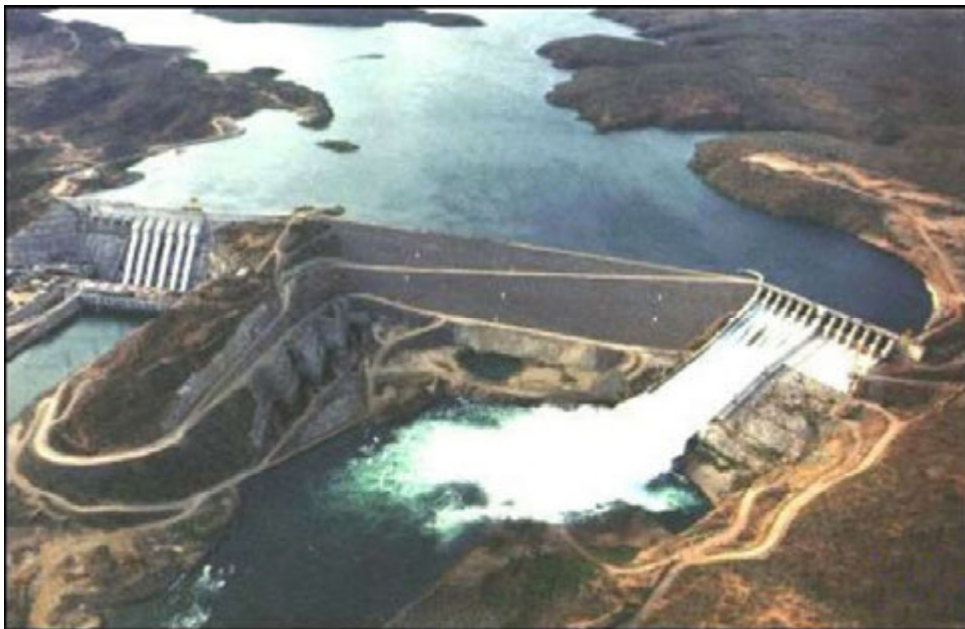
Fig. 10.2 – Xingó Project: service and auxiliary spillway with discharge channel partially lined (Brazil). Discharging capacity 16 500 m 3 /s each one.
