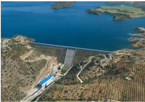
Figure 4.1.- La Breña II Dam (Spain). Gravity RCC dam. (ACUAES)
