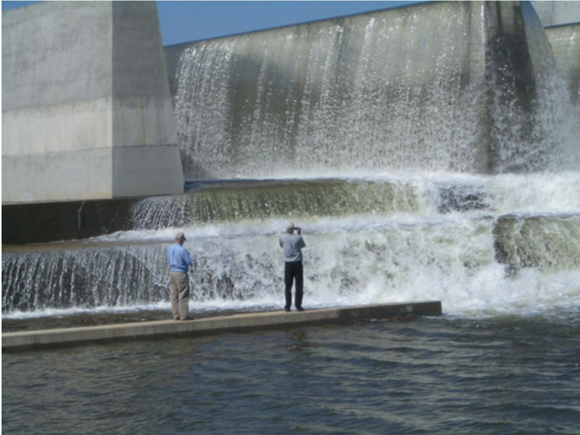
Figure 5.17: Lake Townsend Labyrinth Spillway
