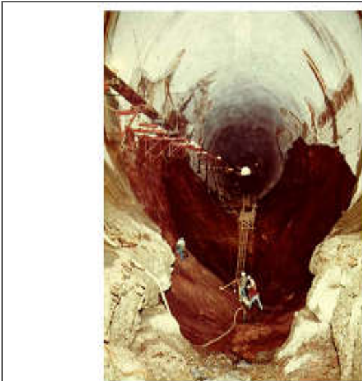
Fig. 7.7 - Damage to Glen Canyon Dam left Spillway in 1983.
