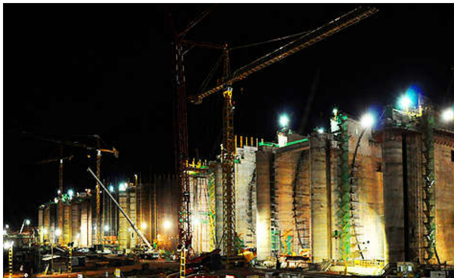
Fig. 2.6 - 82 600 m 3 /s Jirau Project Spillway under construction – Madeira River, Brazil
