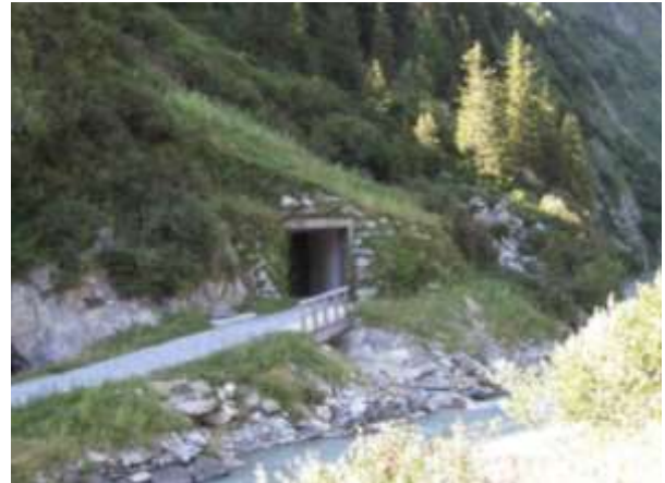
The only remaining visible cavern structure: the access tunnel portal
