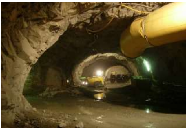
Construction of the storage caverns
