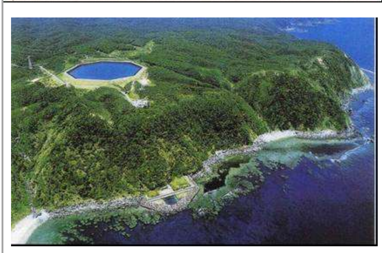
Fig. 8: Kunigami seawater pumped storage plants
