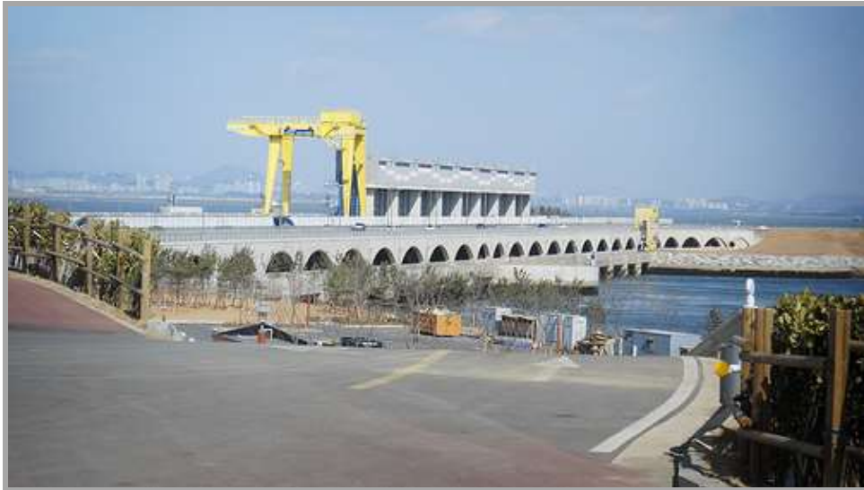
Fig. 24: The Sihwa Lake Tidal Power Station (from Ref. 54)
