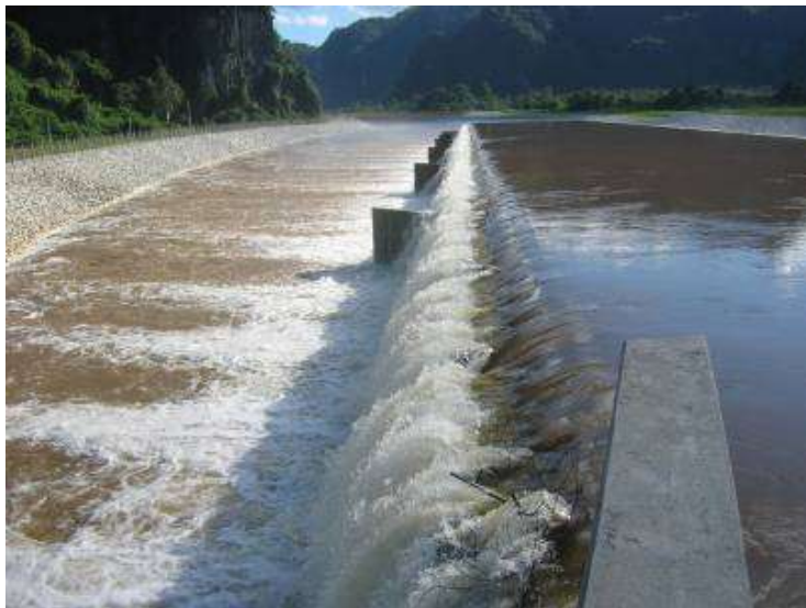
Figure 3 -4: On site view of the aeration in operations for 150 m 3 /s ( EDF)
