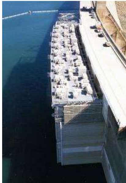
Figure 3-20: Shasta Dam Multi Level Offtake Structure
