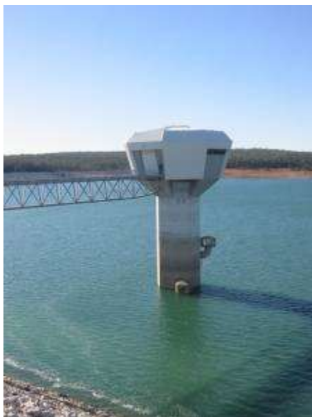
Figure 3-18: Two Intakes Exposed on a Dry Multi Port Intake Tower
