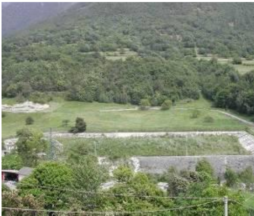
Fig. 3 – Isollaz reservoir before the decommissioning
