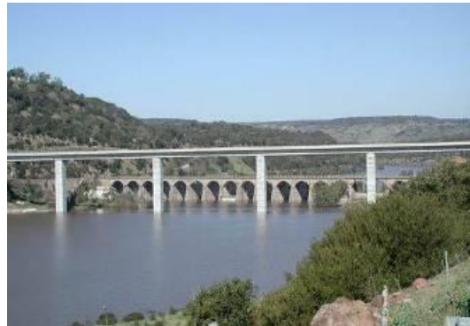
Fig. 8 – Downstream view of the dam: in the foreground the new Omodeo bridge that connects the lake banks
