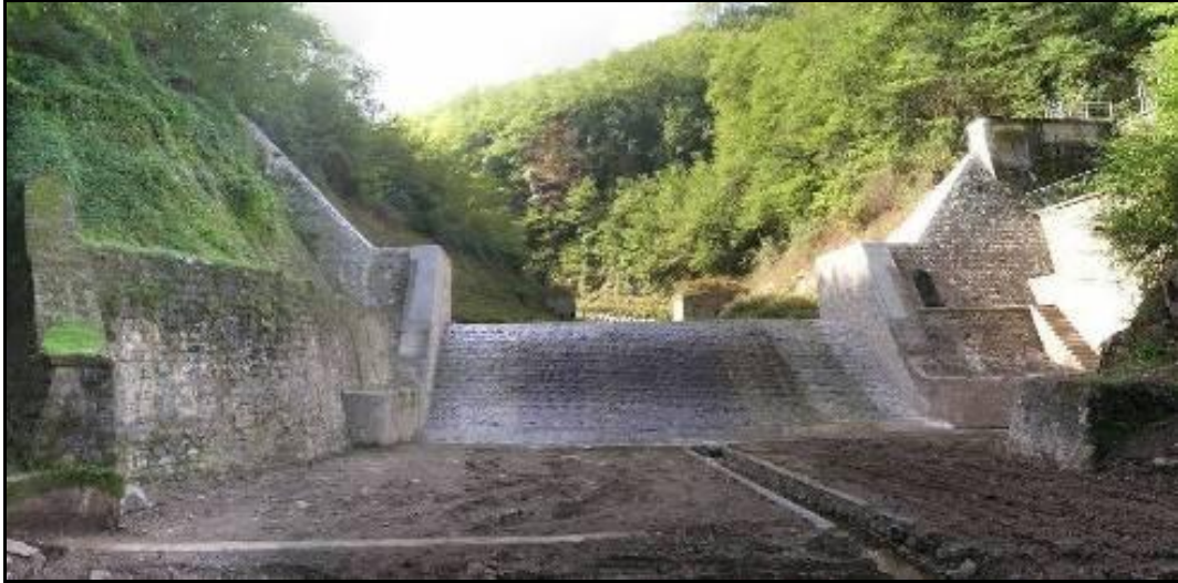
Fig. 10 – The dam after the demolition
