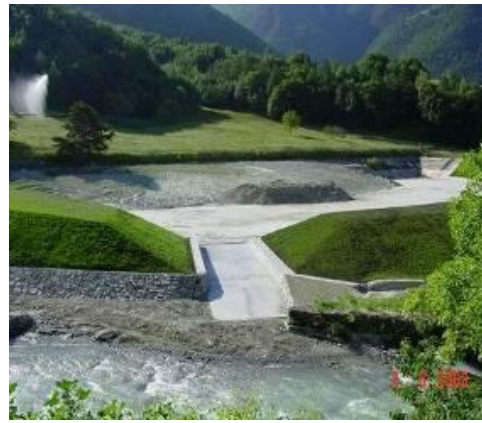
Fig. 4 – View of the actual state of the works
