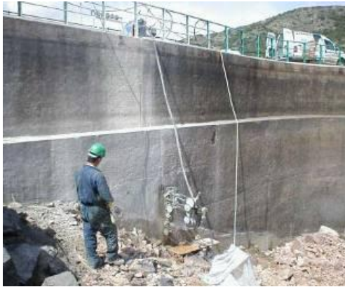
Fig. 10 – The diamond wire cuts and the demolition of the left side of Corongiu dam II to accommodate the new spillway
