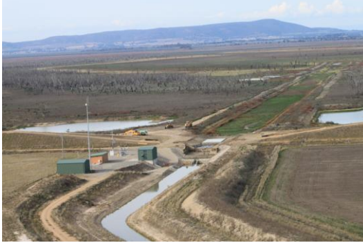
Embankment Breach, Lake Diverters with Pump Station (foreground), Lake Mokoan dry bed (background)
