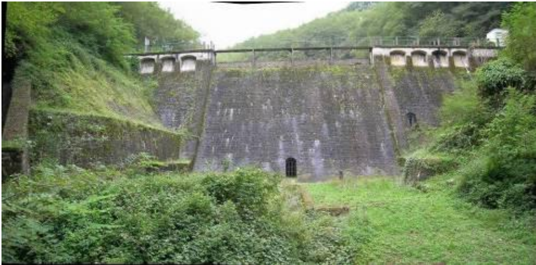
Fig. 9 – The Rio Salita dam before the demolition
