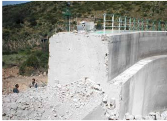
Fig. 10 – The diamond wire cuts and the demolition of the left side of Corongiu dam II to accommodate the new spillway
