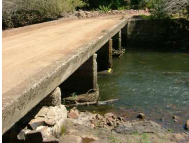
Fig. 8.5 – Type of bridge in the south of Brazil, with a resistant concrete structure, that is able to support high floods underwater.
