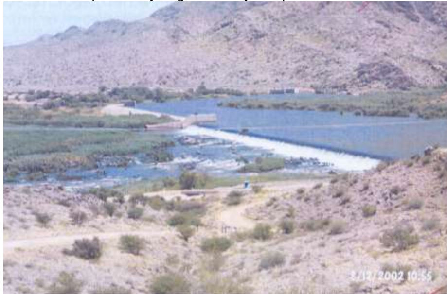
Fig. 2.14 - Photograph of Neusberg weir
