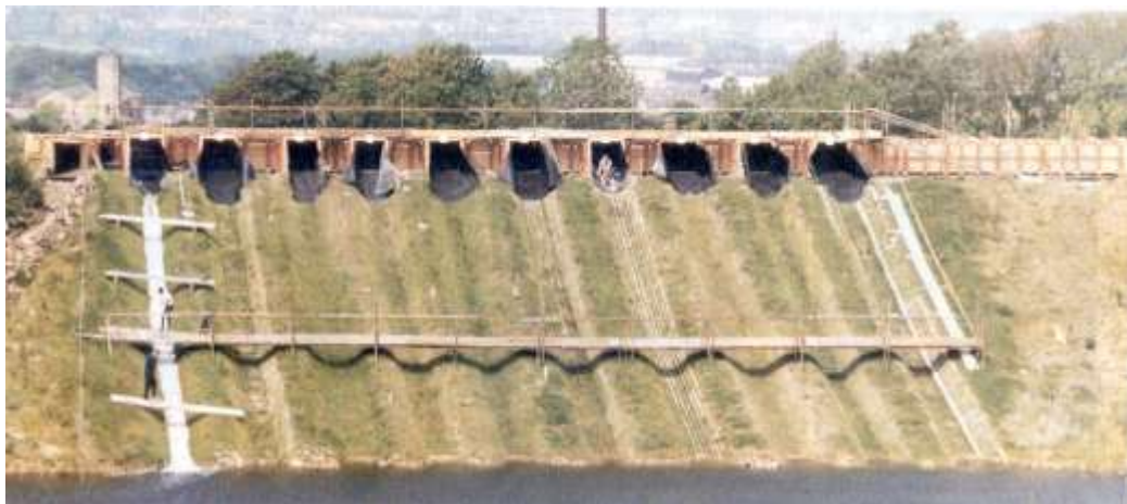
Photograph 7.4: Testing under way on the left-hand of the ten channels at Jackhouse Reservoir near Blackburn, UK
