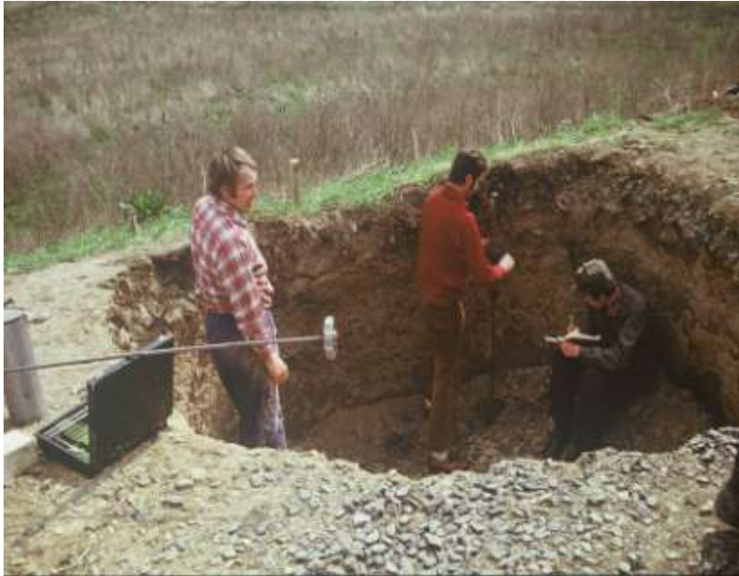
Fig. 3.7 – A sinkhole above failed bottom outlet concrete pipes, in a small dam.
