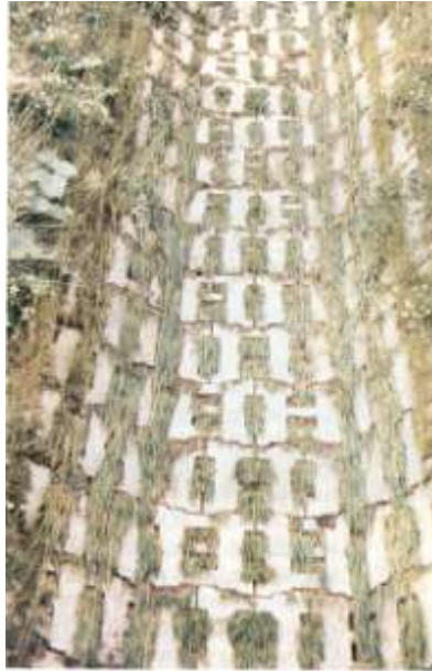
Photograph 7.5: One of the cable-stayed block systems remains totally intact after a water test
