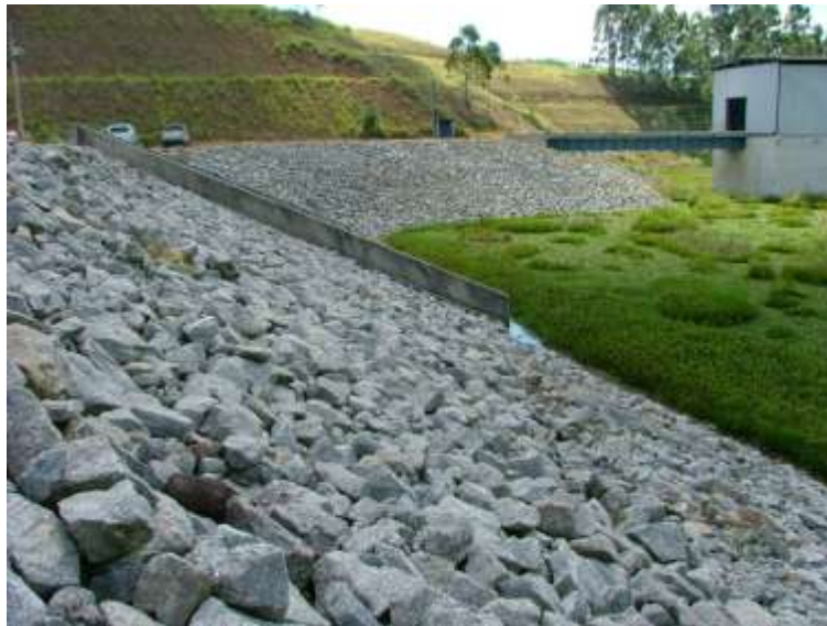
Fig. 5.13: Upstream gneiss rip-rap at the Paraitinga dam, in Brazil.
