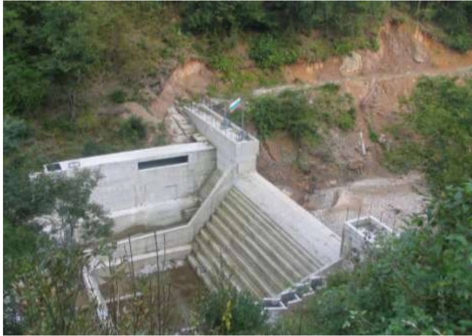
Fig. 2.11 – Lopyan Concrete Gravity dam, 11.60 m height, built in 2004 in Bulgaria.
