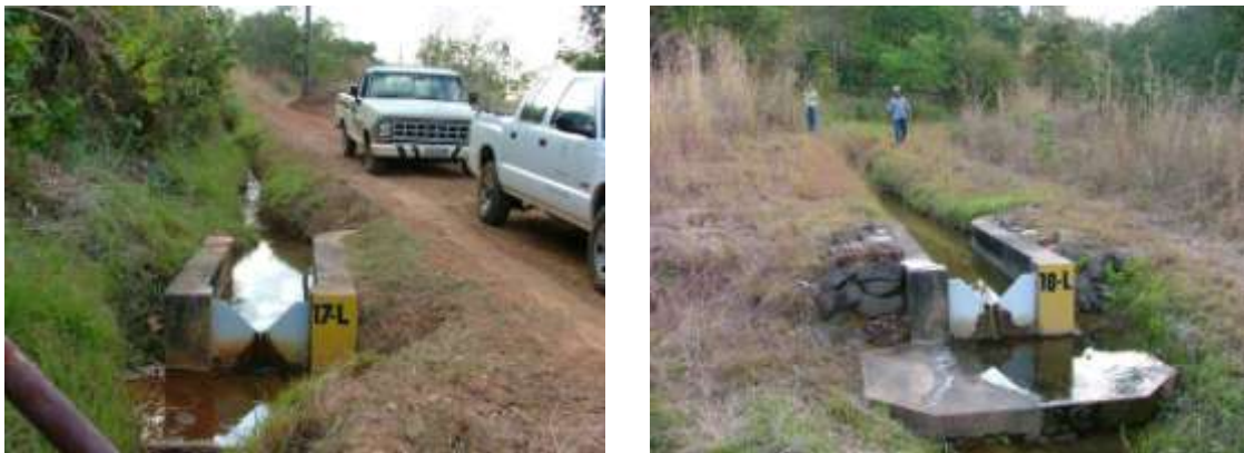
Fig. 6.2 – Leakage measurement using a triangular weir gauge.
