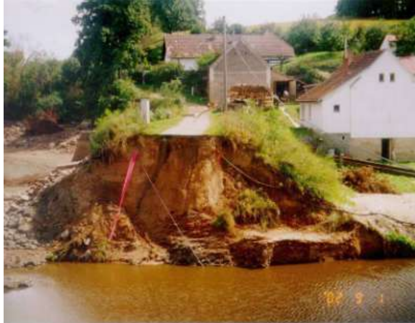
Fig. 3.2 – Massive dam break overtopping, during extremely high floods at the Czech Republic.
