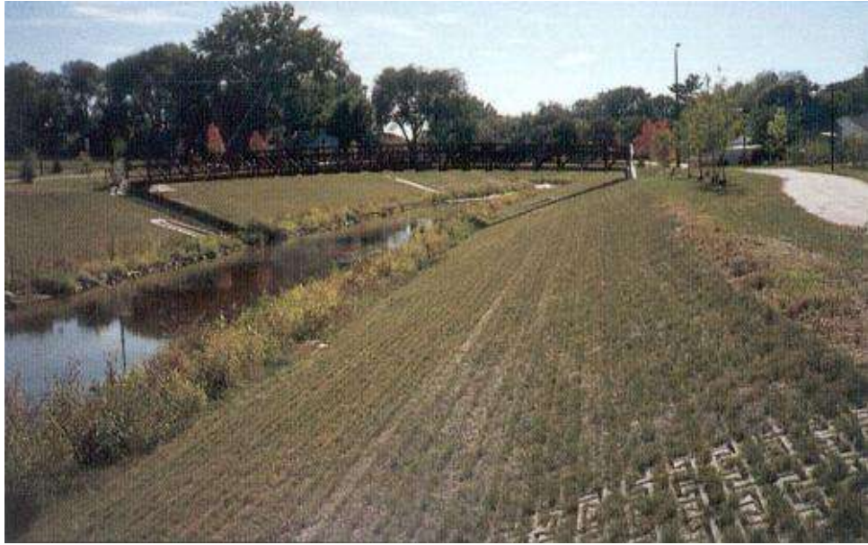
Photograph 7.3: Lateral slopes protected with concrete blocks and grass
