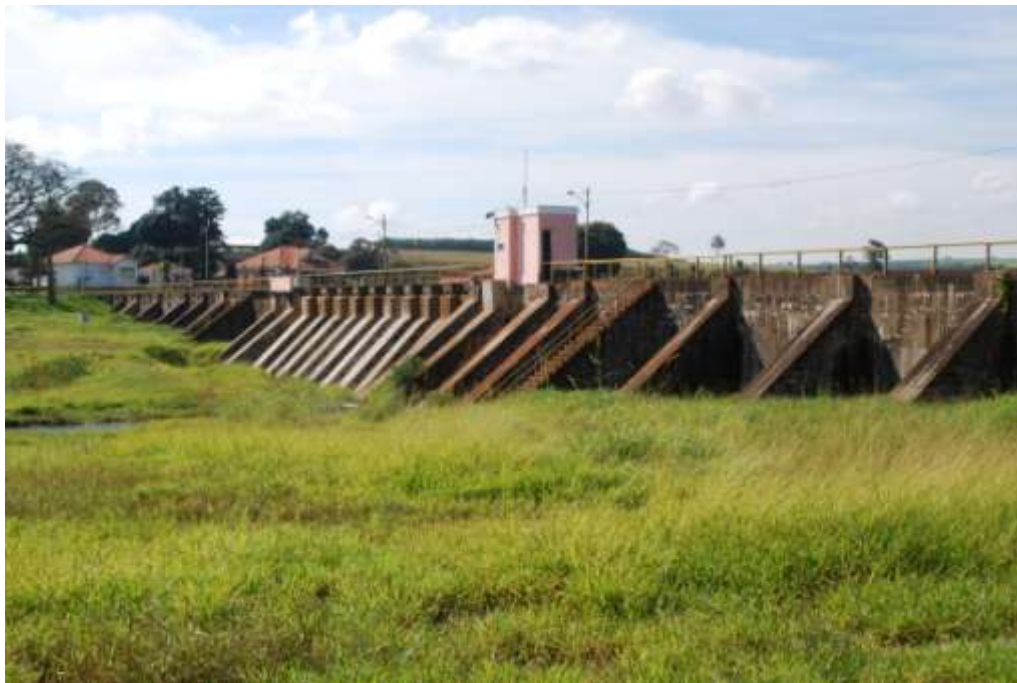
Photo. 2.12 – Barra Buttress Concrete dam, Brazil.
