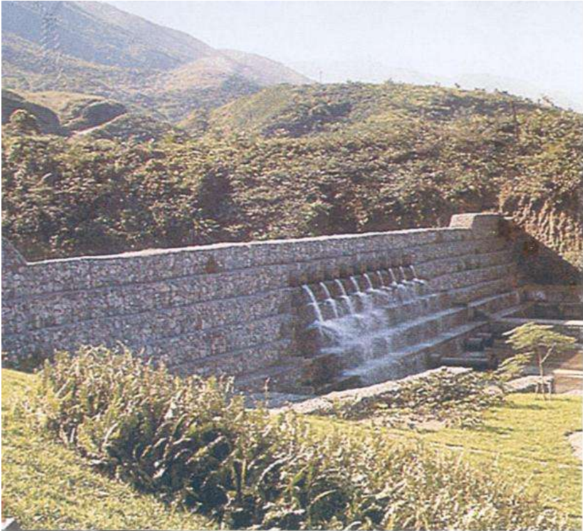
Fig. 2.16 – Gabion dam 12 m high - Brazil
