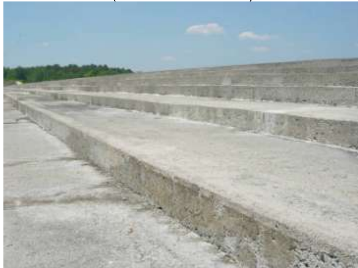
Photograph 7.7: Excellent condition of RCC steps at Tholocco Lake Dam (Abdo and Adaska/07)
