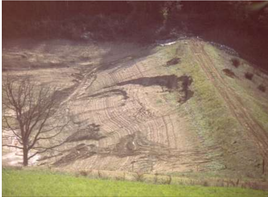
Fig. 3.10 – Sliding of upstream slope of a homogeneous embankment dam after rapid drawdown (France)
