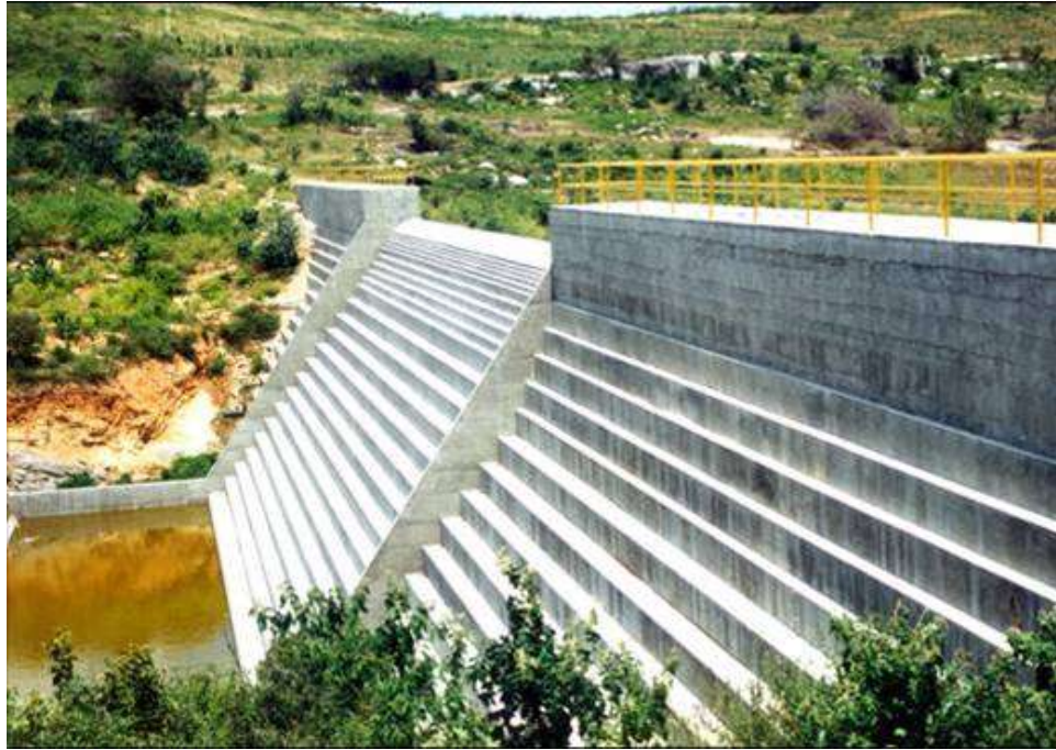
Fig. 2.13 – Trairas RCC concrete dam – Brazil
