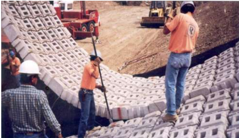
Photograph 7.2: Installation of the articulated concrete blocks in a channel
