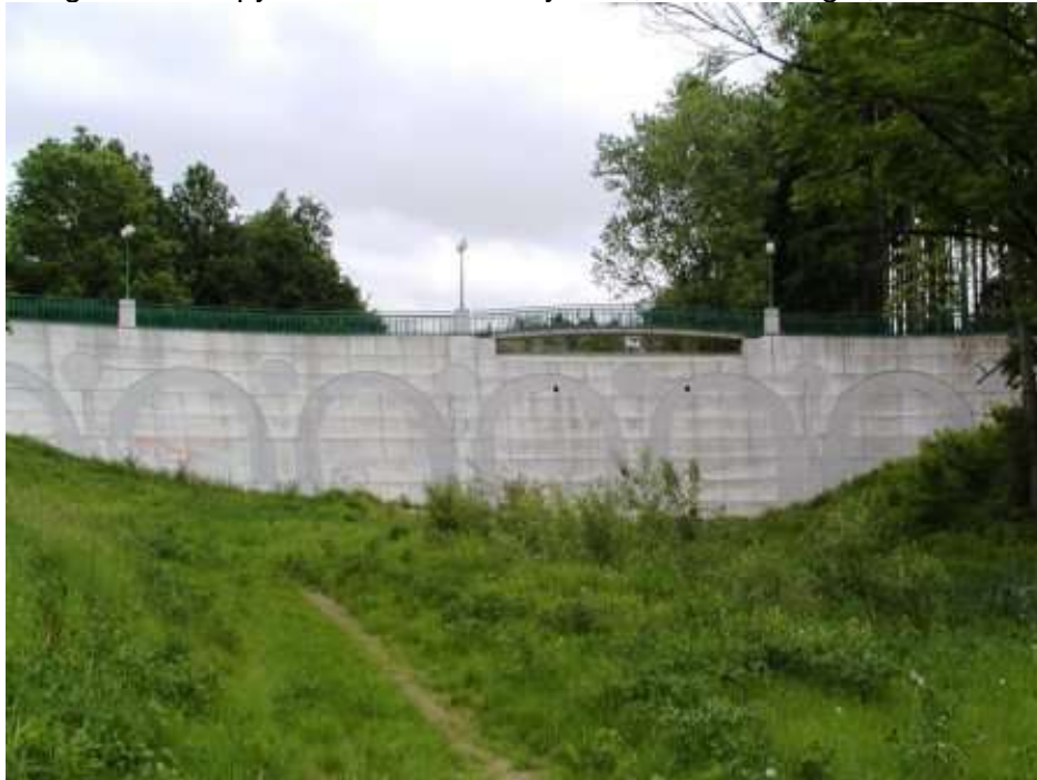
Fig. 2.11a - Hlinky Concrete Gravity dam, height 11m, Czech Republic.
