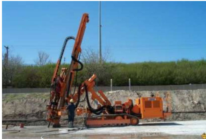
Photograph 7.11: Grout holes are drilled at optimized angles for rock joints patterns (image from www.advancedconstructiontechniques.com/ ).
