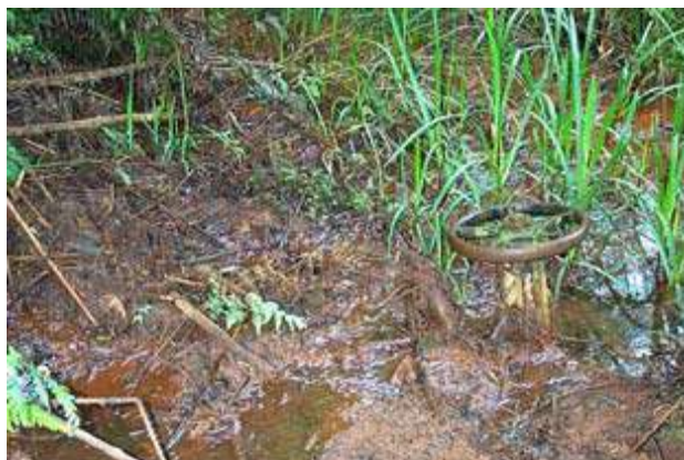
Photograph 7.16: What are the chances that this valve will work in an emergency? (SMEC/2006)
