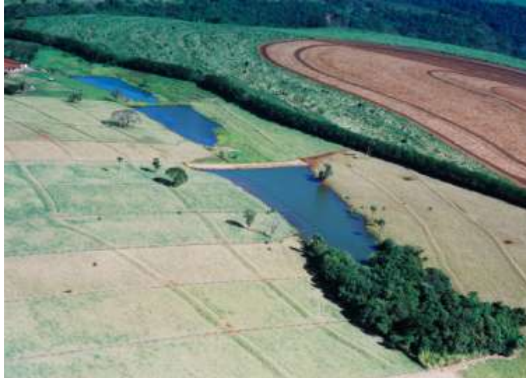
Fig. 8.1 – Three small dams in cascade along a farm river, in Brazil.
