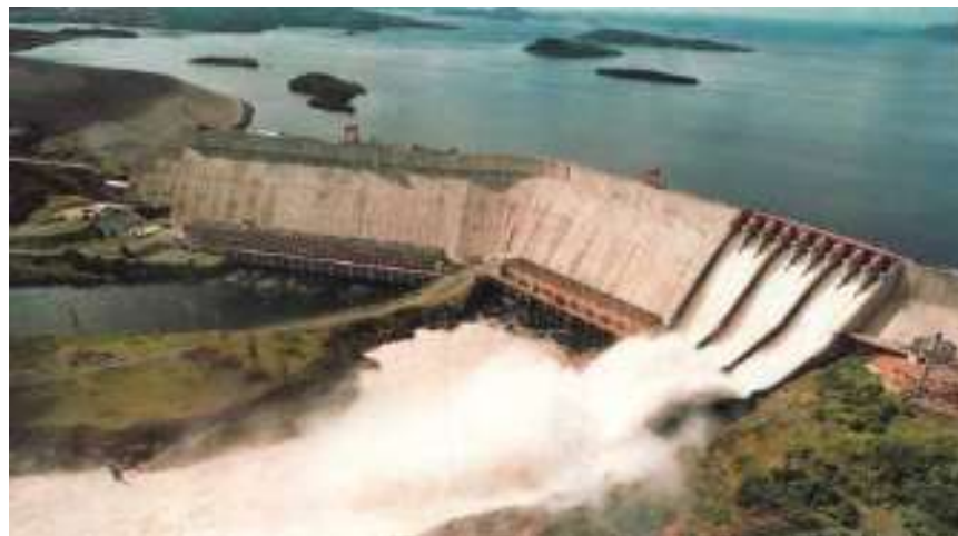
Figure 7.4- Guri Dam, Venezuela
