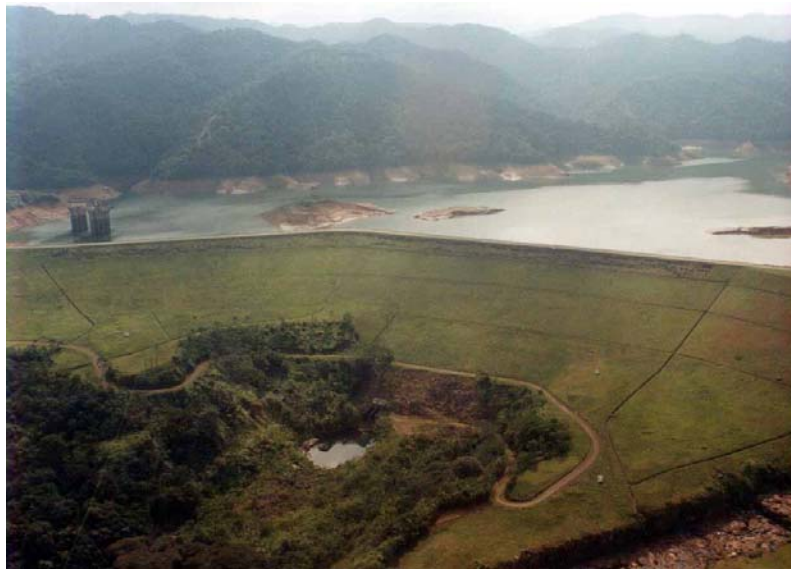
Figure 8.2- General Overview of Punchiná Dam
