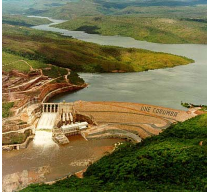
Figure 7.3- Corumbá I Earth Core Rockfill Dam, Brasil.
