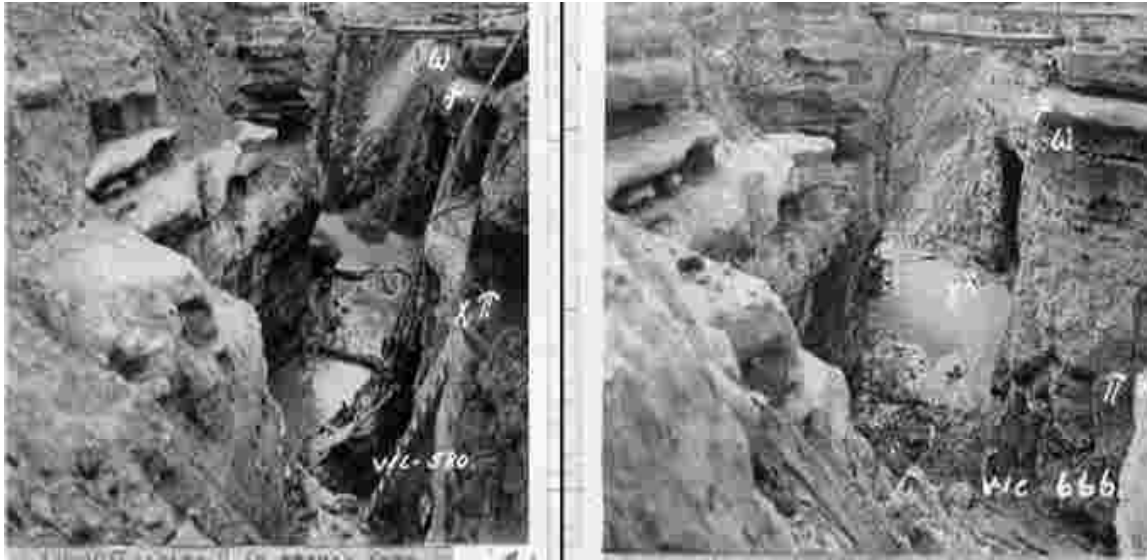
Fig. 4 Before and After Photos Showing Trench Clean-up
