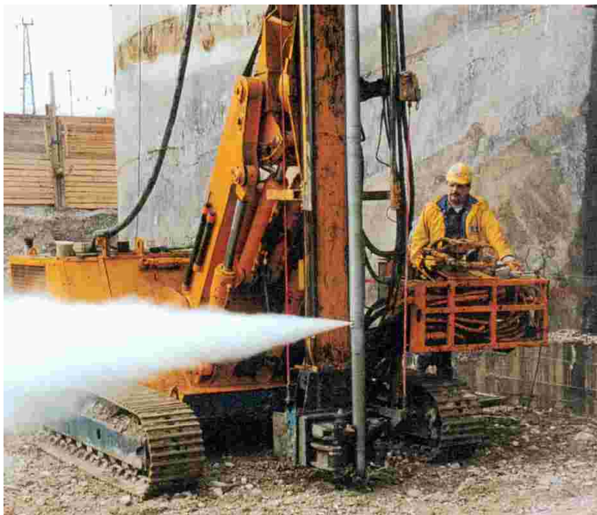
Fig. 7.1 Jet grouting rig in operation above ground
