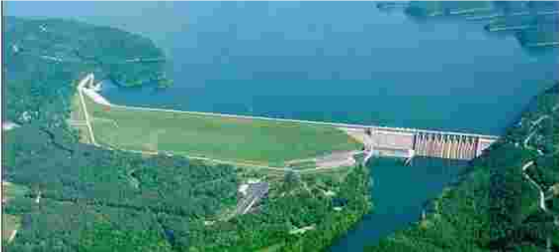
Fig. 1 Aerial Photo of Wolf Creek Dam
