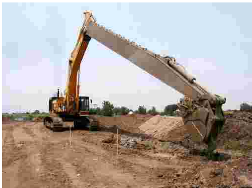
Fig. 3.16 Long-stick backhoe excavator
