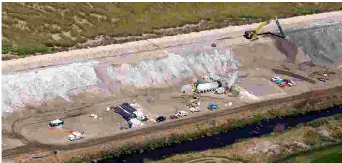
Figure 5: Aerial photo showing CB wall excavation approaching the slurry plant
