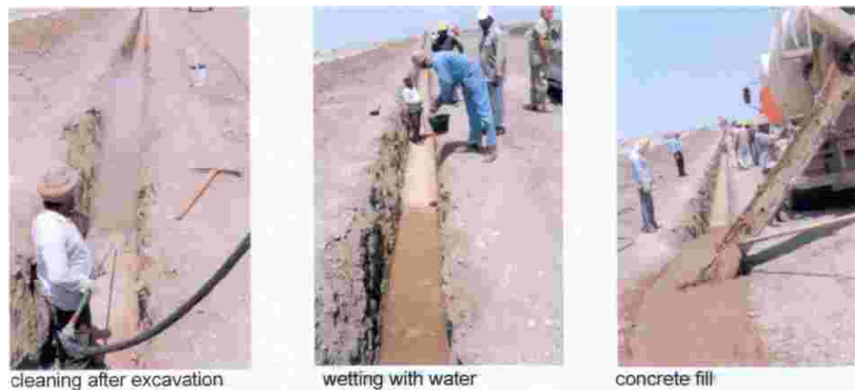
Fig. 3.1 Plastic concrete wall construction in Wadi Tanuf (Sultanate of Oman)
