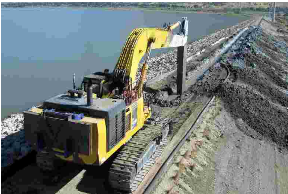
Figure 6: Photograph of typical CB cutoff wall excavation through the dam crest
