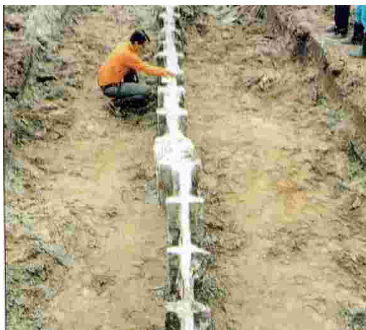
Fig. 4.2 Partly excavated Vib-wall at Lake Altmühl (Germany)
