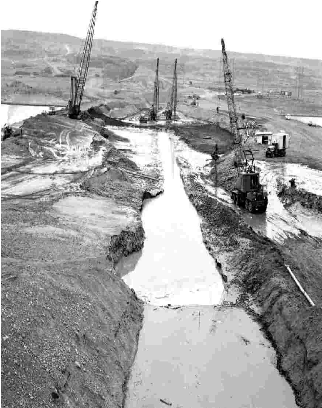
Figure 5 Slumped slurry trench, note use of draglines and clam-shell excavators
