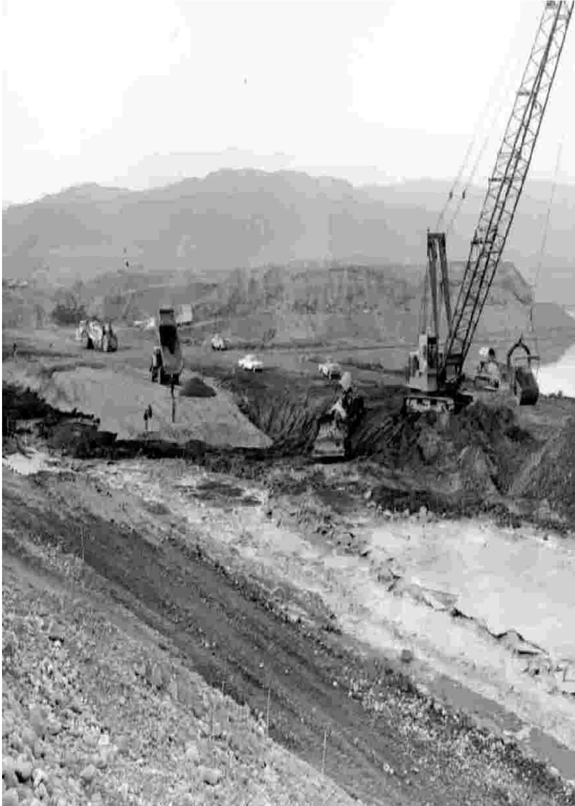
Figure 6 Fill placement, cleaning, and repair of slumped slurry trench
