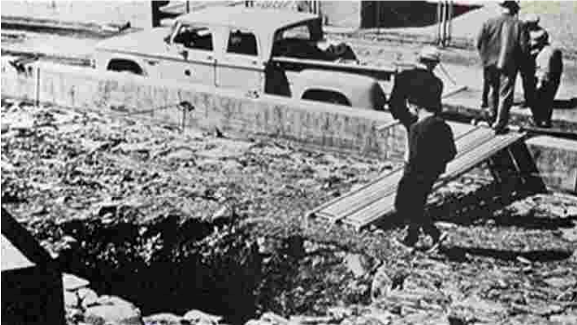
Fig. 5 1968 Sinkhole in Toe of Embankment above Switchyard
