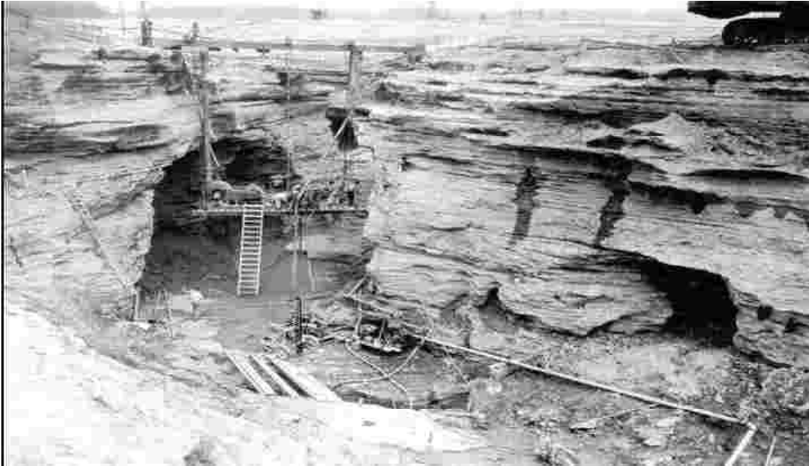
Fig. 3 View of Solution Channel/Cutoff Trench
