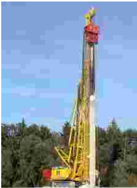
Fig. 3 Crawler crane SW 311 with hydraulic vibrator MS 200 H
