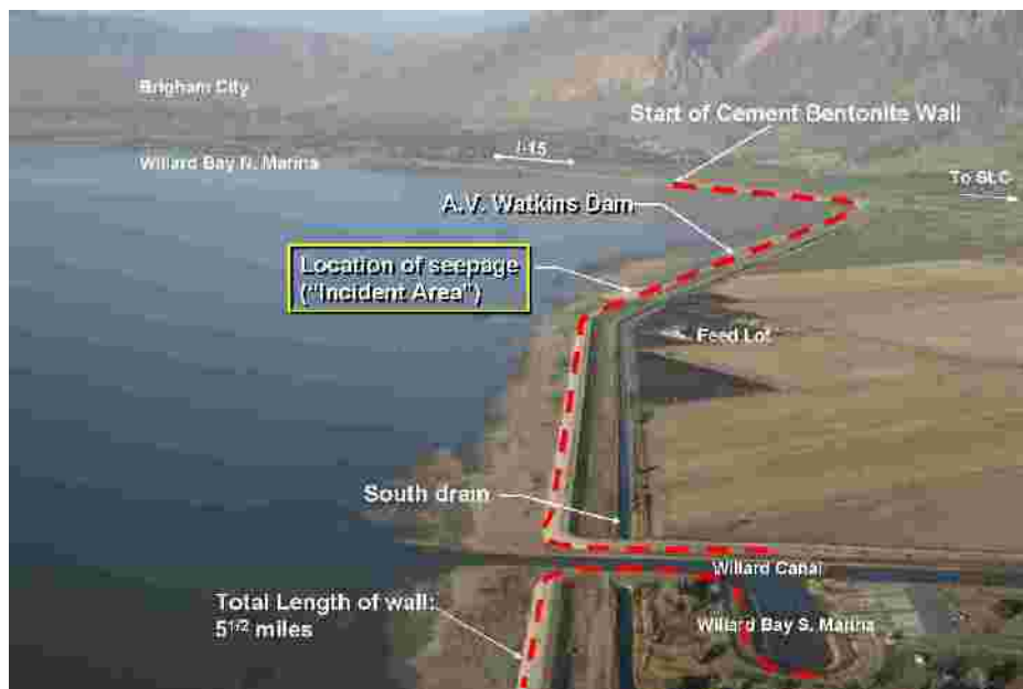
Figure 4: Aerial photo showing alignment of CB cutoff wall through the south eastern portion of the dam, including the section that nearly failed (incident area)
