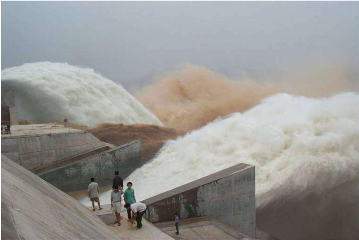
**Figure 5.11-10 Xialongdi Dam, China, during commissioning test**
