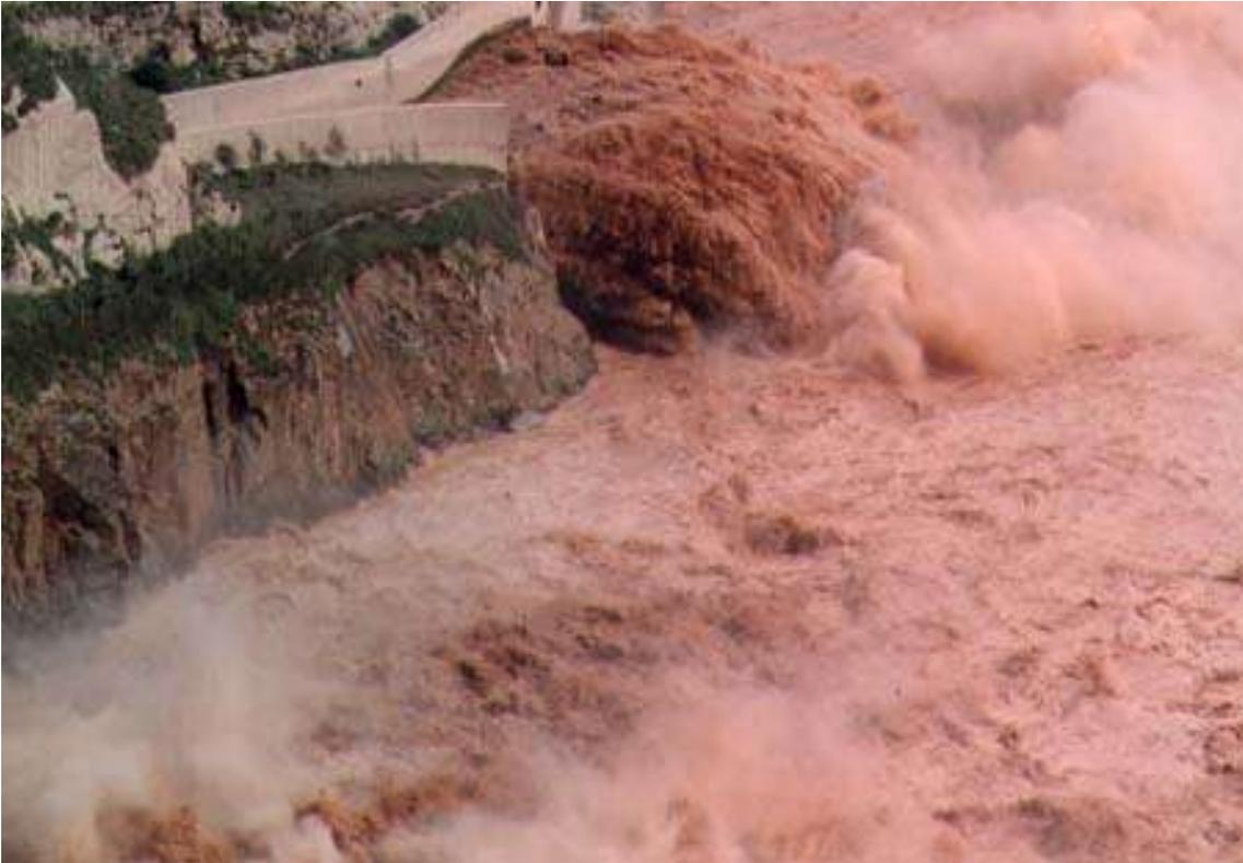
**Figure 3.10-8 Sediment flushing at Sanmenxia Dam (side outlet)**
