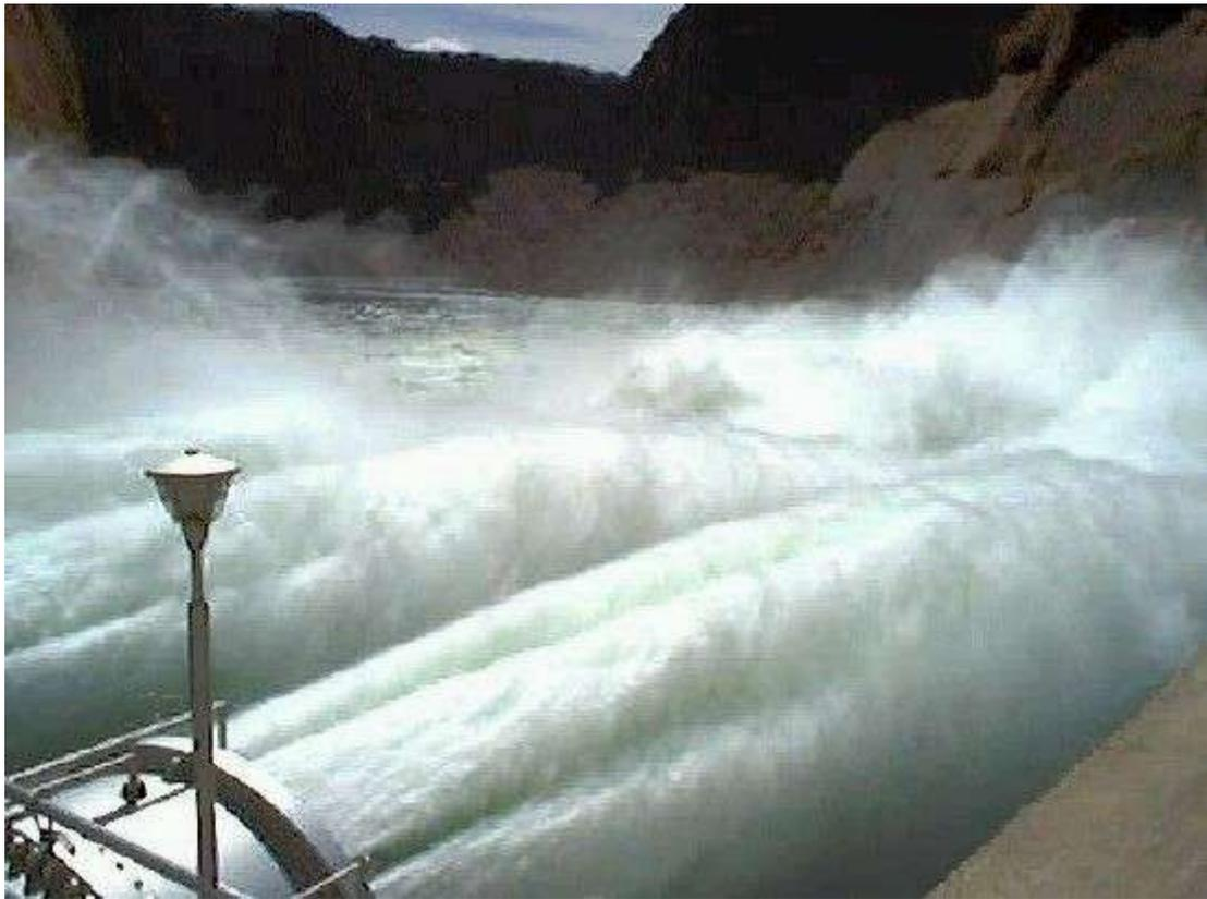
Figure 3.10-2 Glen Canyon Dam 1275 m<sup>3</sup>/s flood release (USGS, 2002b)
