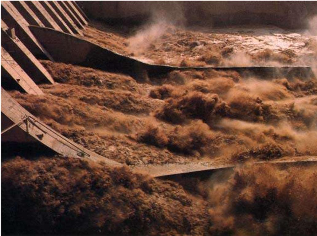
**Figure 2.1-2 Sanmenxia Reservoir flushing after reconstruction of the outlets**
