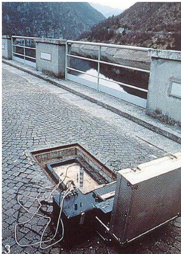
Fig. 6.10 – Thermal measurements on concrete at a dam
