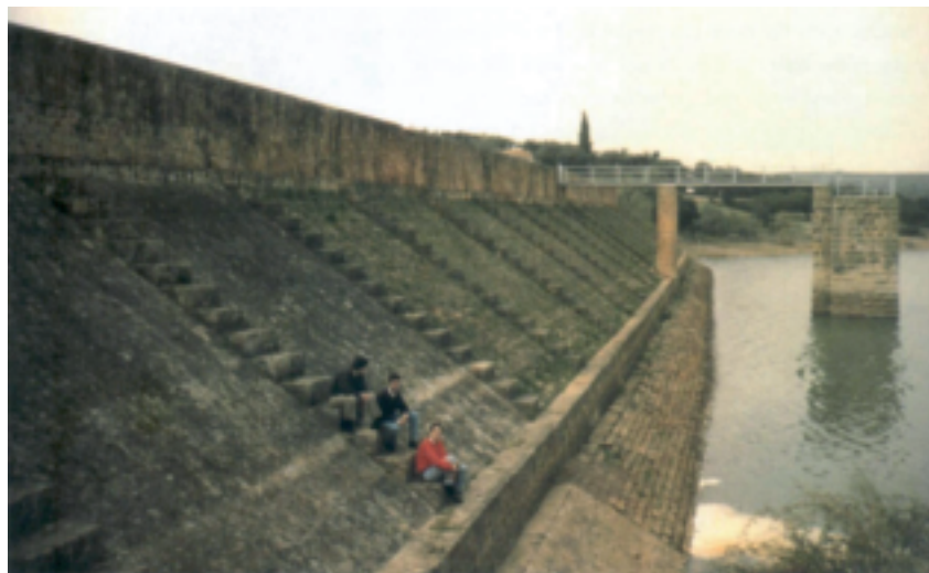
Fig. 63 The Roman Dam of Cornalvo (Mérida) reconstructed at the beginning of the 20th century (Arenalles/2006)
