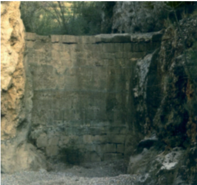
Fig. 67 El Galindo Dam (15th century) in Blesa – Zaragoza (Arenillas/2006)
