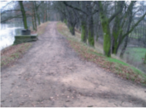
Fig. 20 Stebensky pond dam built in 1720, with 7,6 m height and 180 m long
