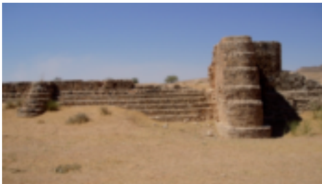
Fig. 46 DS Megenin dam downstream view of buttresses and steps
