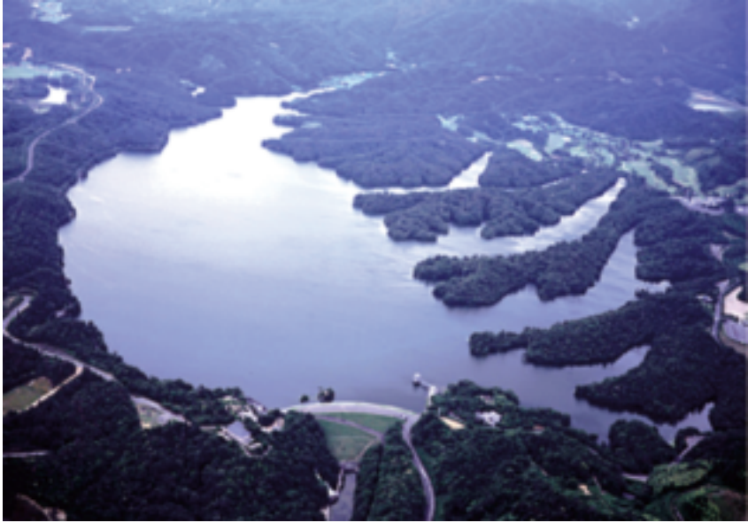
Fig. 40 Overview of Mannoh-ike: Mannoh-ike Land Improvement District (Kagawa Prefecture) (Largest Tameike in Japan, Dam height 32 m, Reservoir volume 15 400 000 m 3 )
