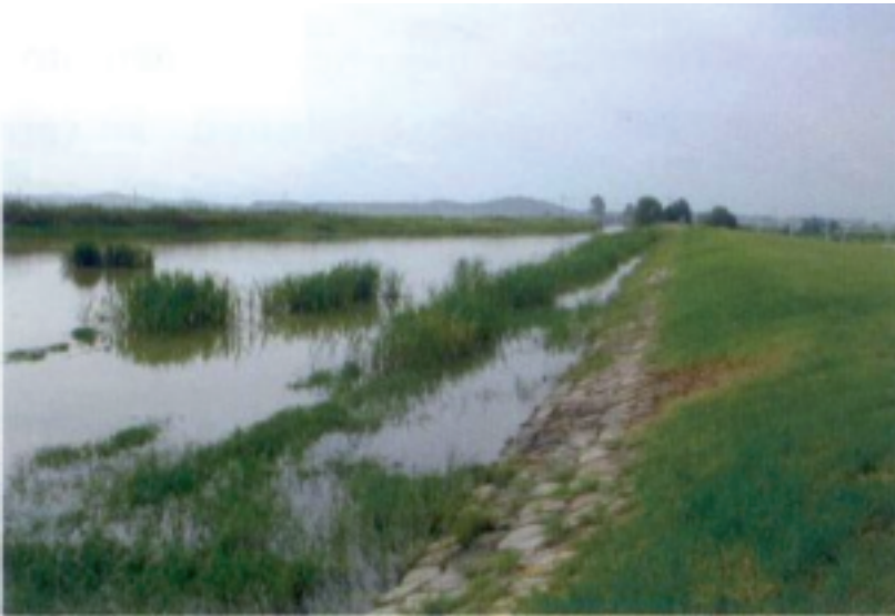
Fig. 42 View of reservoir and dam slope, in Korea
