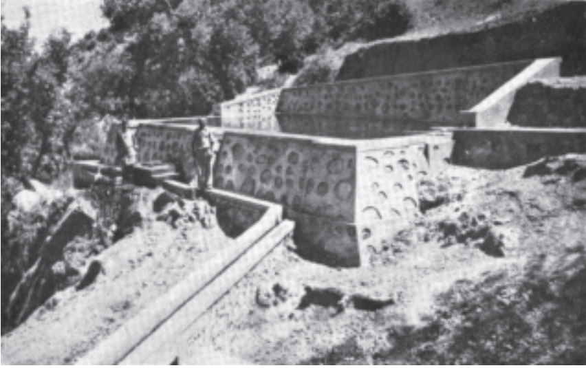
Fig. 15 Masonry reservoir and intake channel
