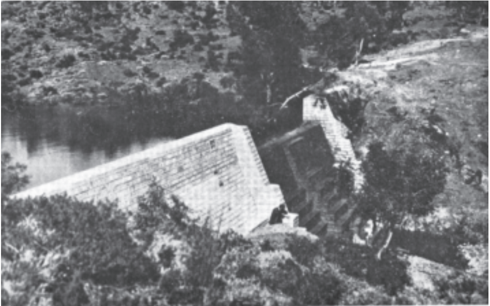
Fig. 14 The Kophinou masonry dam
