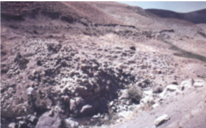
Fig. 75 Upstream dam on Doni creek
