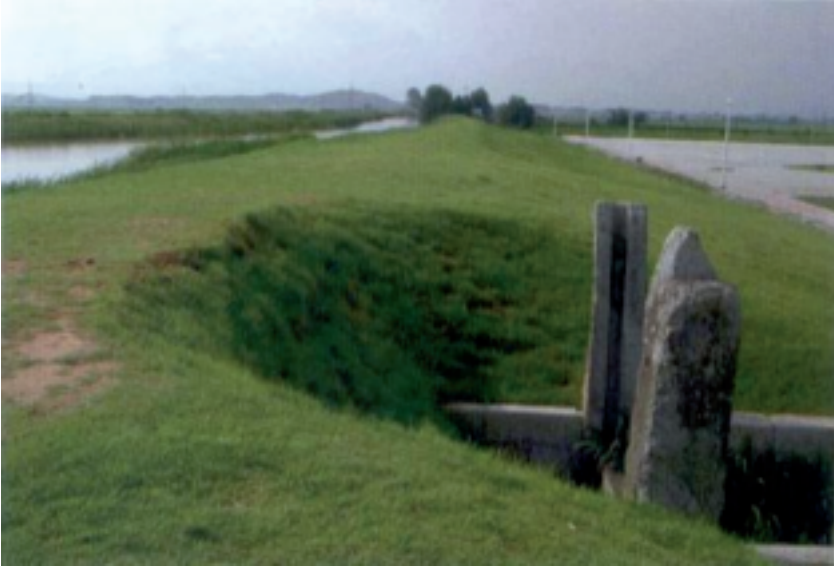
Fig. 43 Dam itself and water gate of Byeoggolje, Korea
