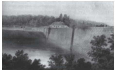
Fig. 26 Saloupe Dam: upstream facing
