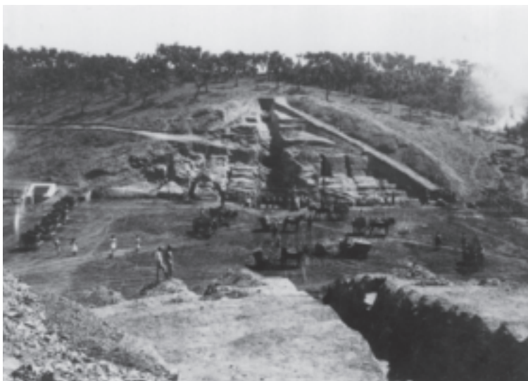
Fig. 52 Excavation of the drainage and cutoff trenches [1]
