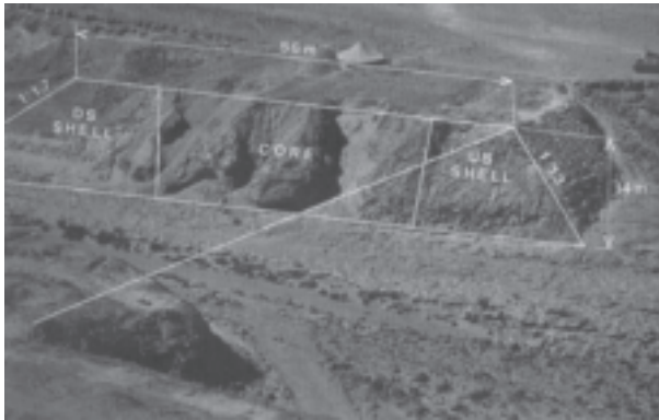
Fig. 1 View of Kafara dam site from the left bank (Schnitter/94)
