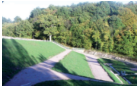
Fig. 24 Torcy-Vieux dam : downstream face after year 2000 reinforcement
