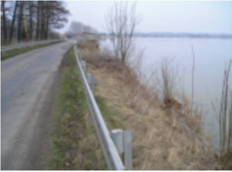
Fig. 18 Vavrinec pond earth dam built in 1480, with 8,0 m height and 380 m long
