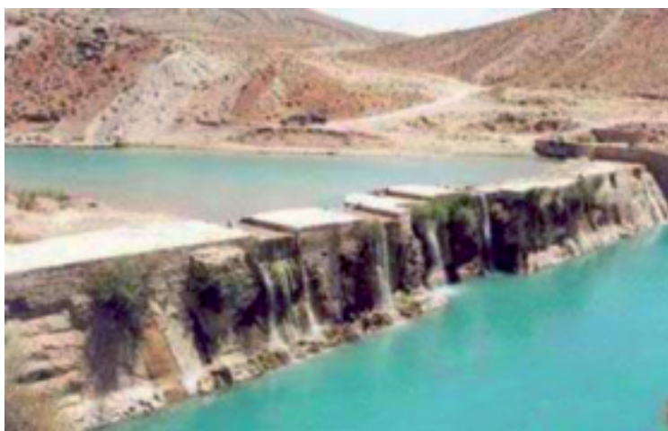
Fig. 33 Bahman dam 8 m high and 117 m long built ~2000 years ago
