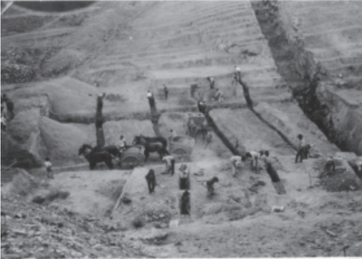
Fig. 50 General view of the Fontes dam during its construction, in 1937. [1]
