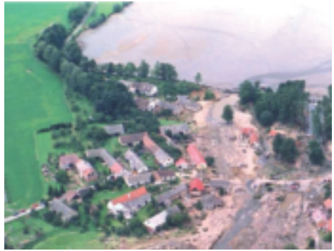
Fig. 21 Metelsky pond plane view during catastrophic flood at 08/2002 (dam was damaged)
