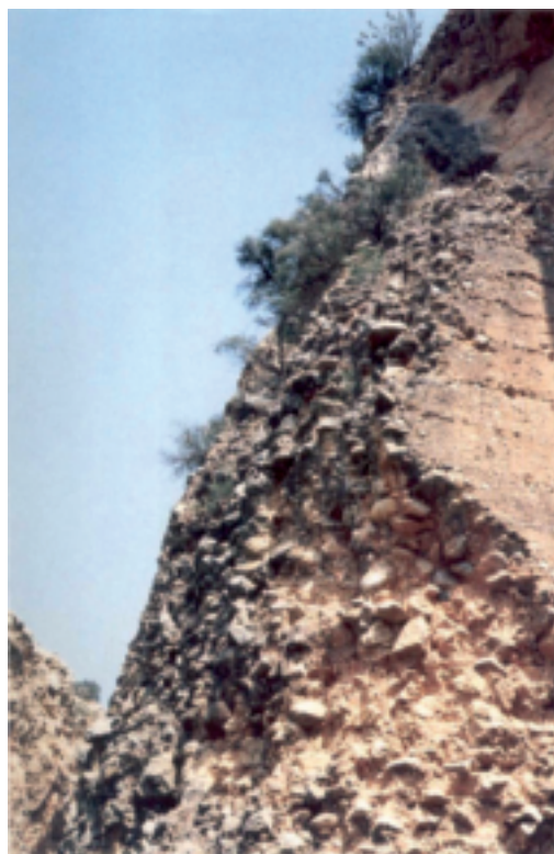
Fig. 66 Remains of the right abutment of the Malpasillo Dam - 14th century (Arenalles/2006)
