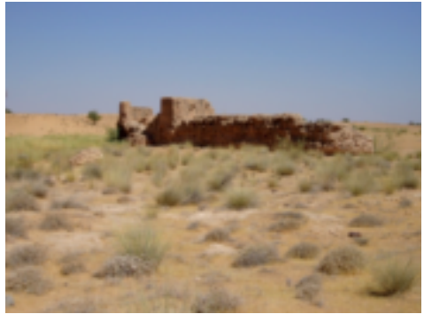
Fig. 45 General view of the DS Megenin dam
