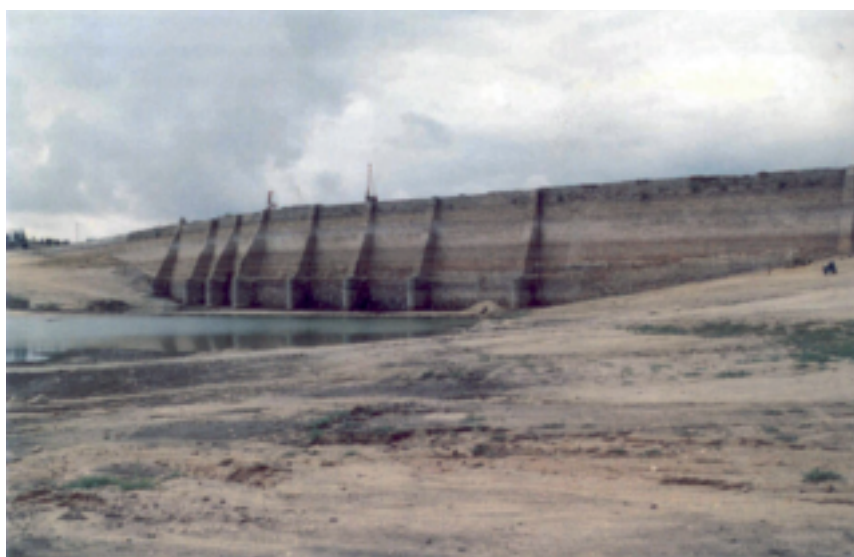
Fig. 61 The Roman Dam of Proserpina from upstream in 1992 (Arenillas/2006)
