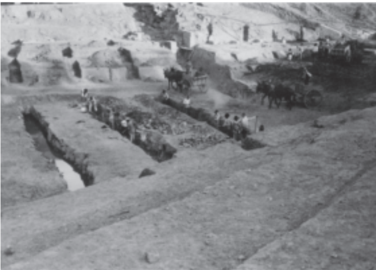
Fig. 51 First stage of the earthfill compaction at the river channel [1]
