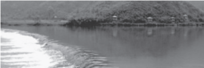
Fig. 11 Tongjiyan Dike built in 502~519 A.D., first arch dam known.
