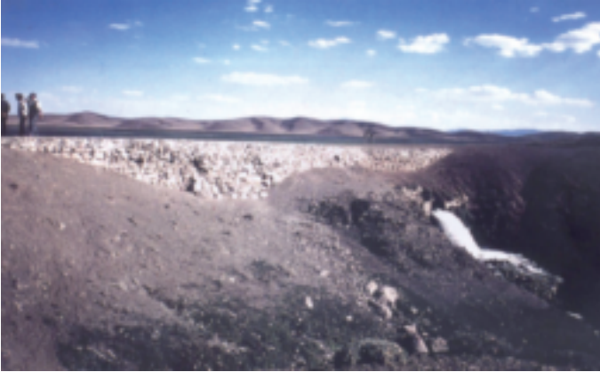
Fig. 74 The 5.4 high northern dam at Kesis lake, upstream of the initial dam site, and discharge from the bottom outlet
