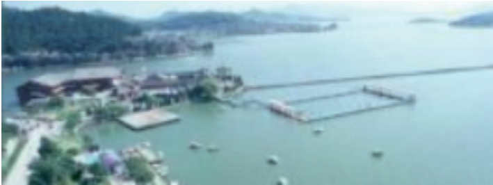
Fig. 10 Dongqian Lake Embankment built in 744 A.D., with a length of 45 km
