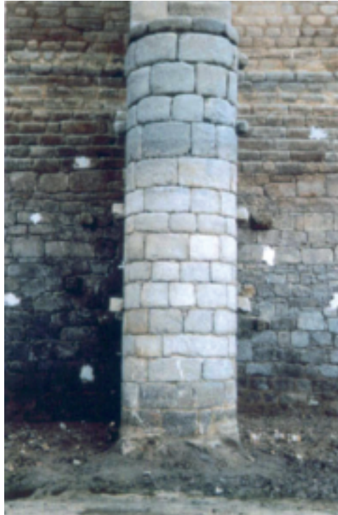
Fig. 62 Proserpina Roman Dam (Mérida): Detail of a buttress (Arenillas/2006)
