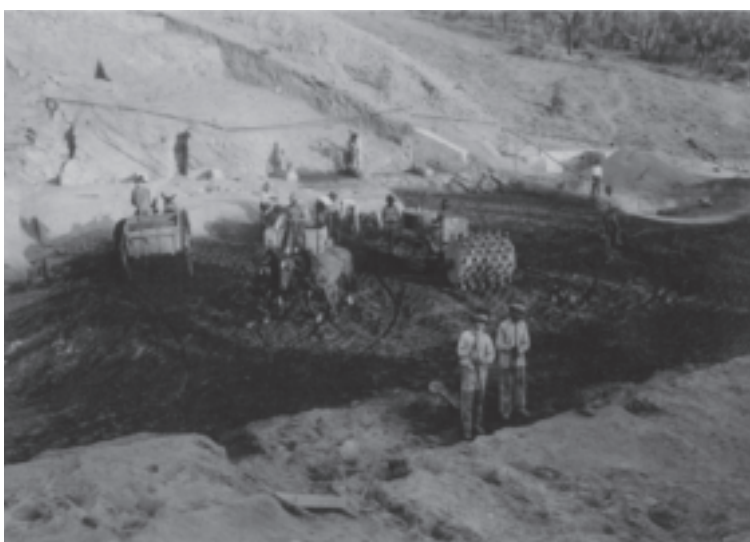
Fig. 53 Detail of the drainage trenches excavation, downstream the cutoff [1]
