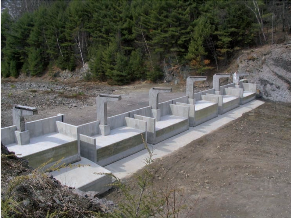
Fig. 8 Concrete fuse plug, Terminus Dam, California, USA
