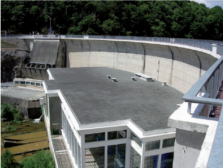
Fig. 3 Mervent dam in France
