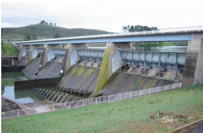
Fig. 7 Gated Spillway, Scrivener Dam, Canberra, Australia
