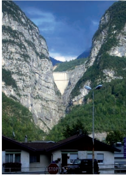
Fig. 2 Vajont arch dam in Italy
