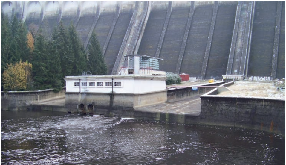
Fig. 9 Low-level Outlet, Eupen Dam, Belgium
