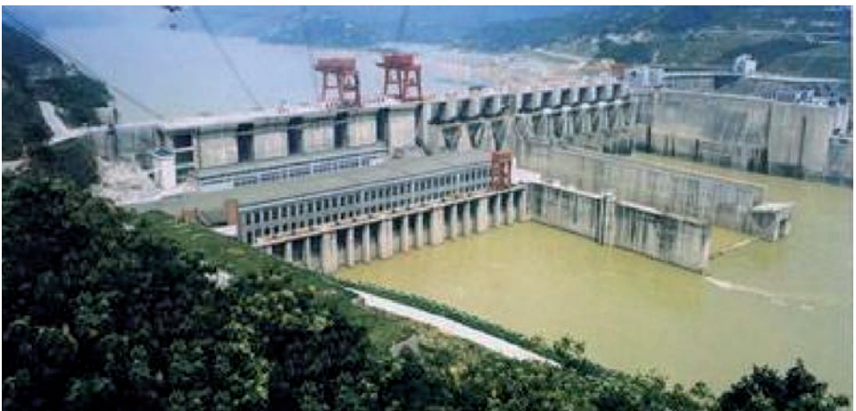
Fig. 18 Wuqiangxi Dam and HPP China
