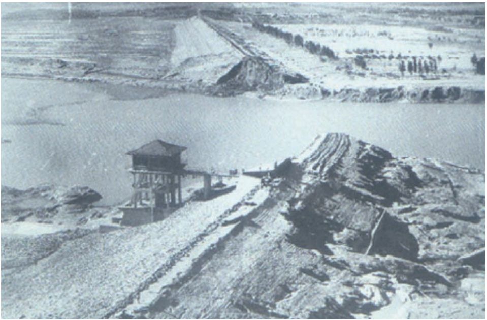
Fig. 16 Banqiao Dam (Ruhe River, China) after the break
