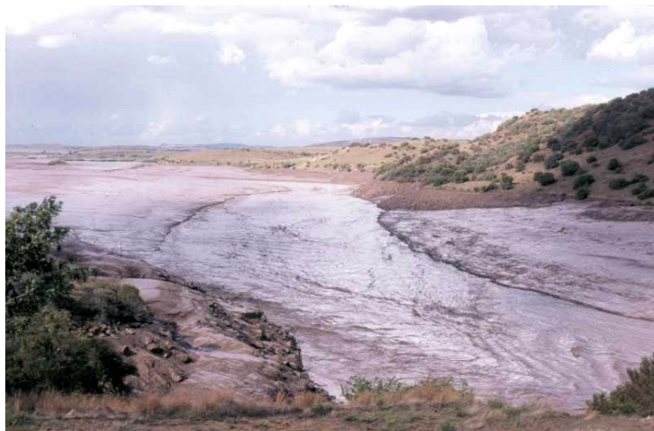
Figure 5.2-9. Welbedacht Reservoir during flushing
