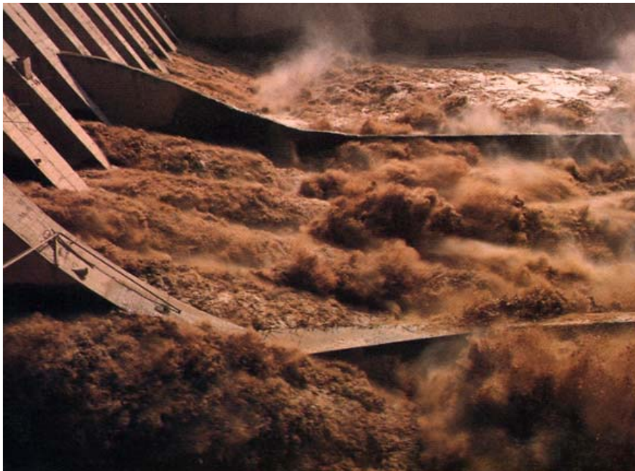
Figure 2.3-2. Sanmenxia Reservoir flushing after reconstruction of the outlets
