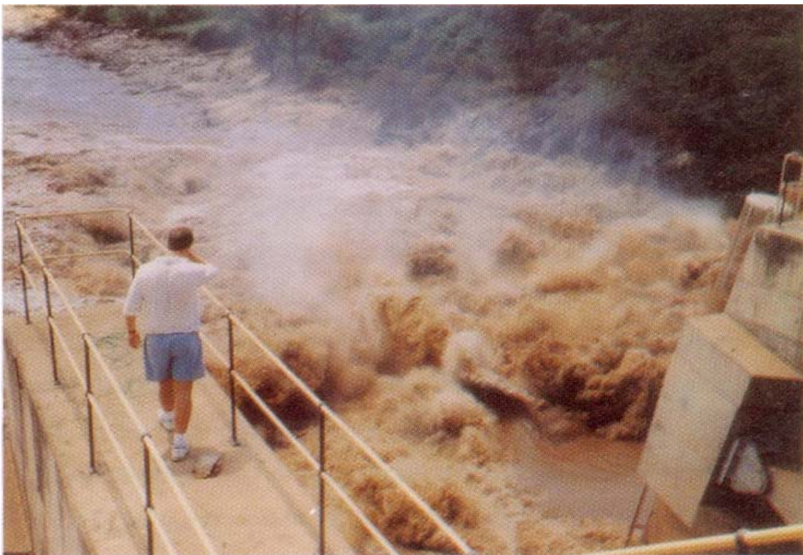
Figure 5.1.2-1 Phalaborwa Barrage flood flushing (900 m 3 /s, February 1996)
