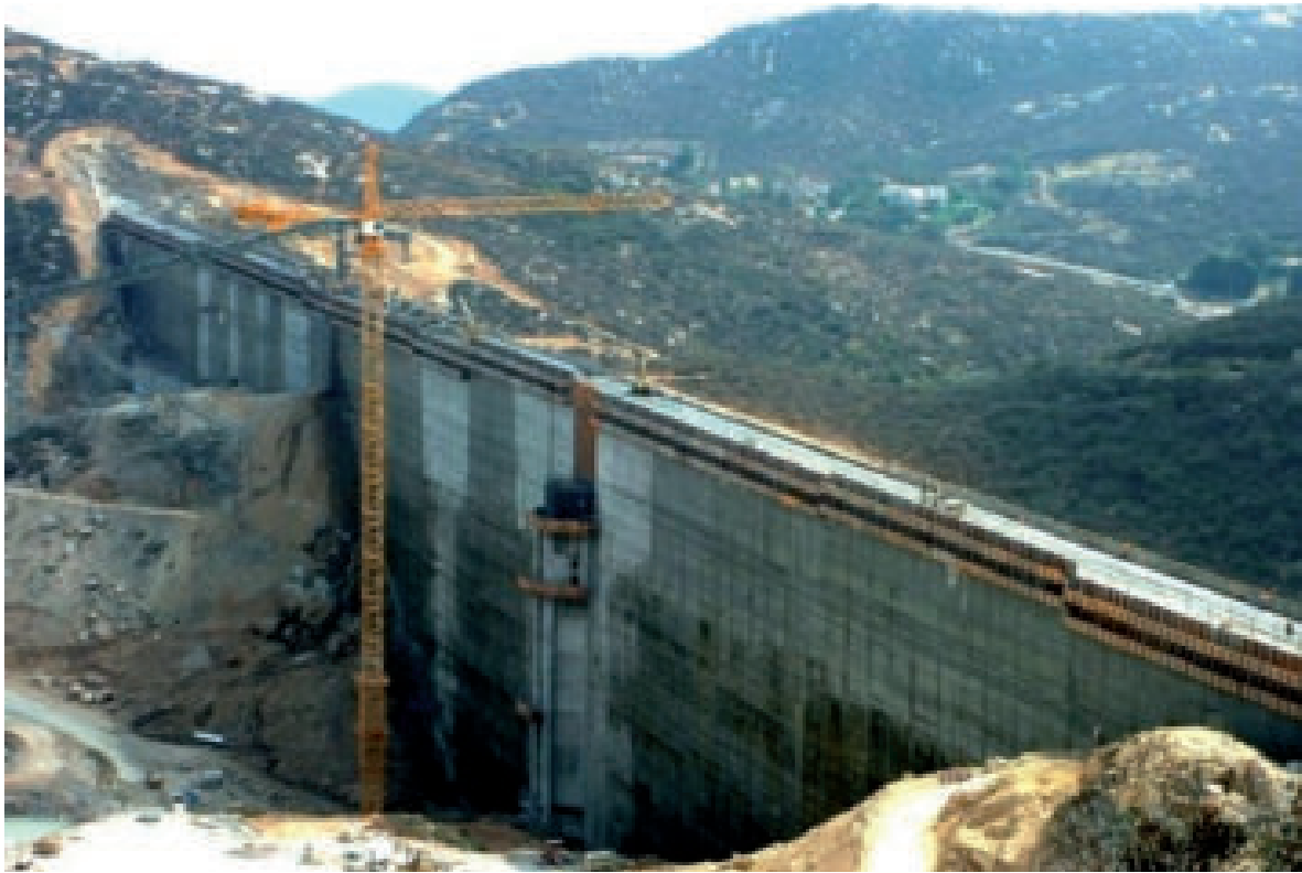
Fig. 12 Olivenhain Dam at Approximately 97% Completion
