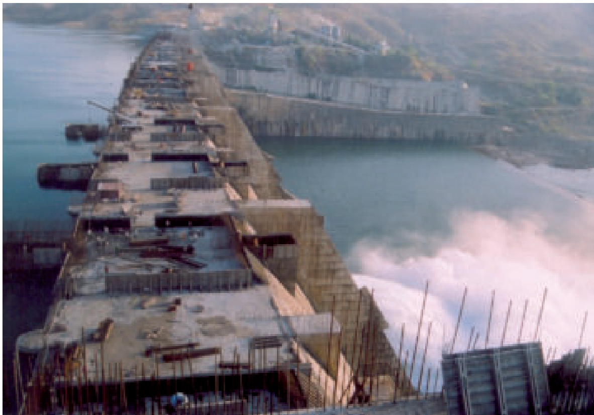
Fig. 7 Sardar Sarovar dam under construction
