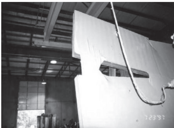
Fig. 123 Destructive testing of Penn Forest panel
