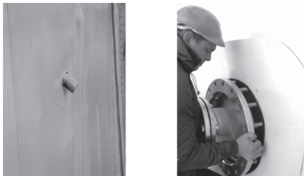
Fig. 60 and 61 Watertight connections at synthetic pipe and steel pipe
