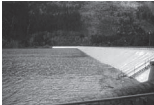
Fig. 64 Moravka, Czech Republic 1999, PVC geocomposite sheets anchored at 6 m spacing
