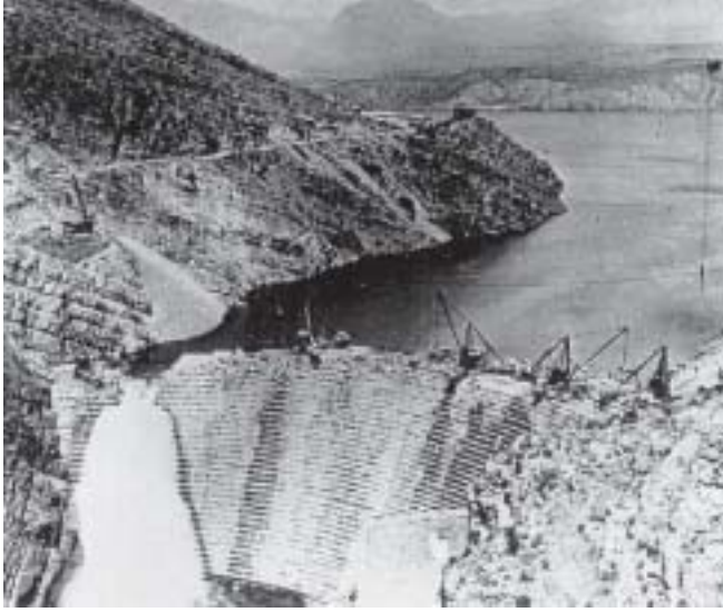
Fig. 6.35. Theodore Roosevelt dam during the original construction Barrage Theodore Roosevelt pendant la construction
