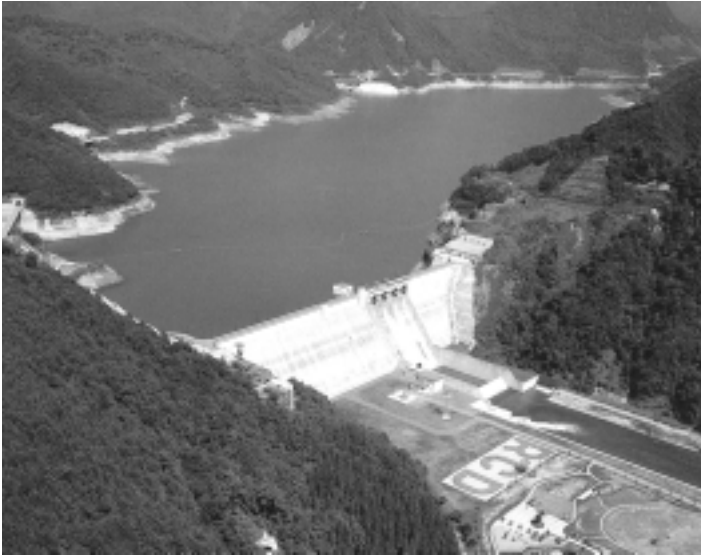
Fig. A-2.1 Photograph of Tamagawa dam
