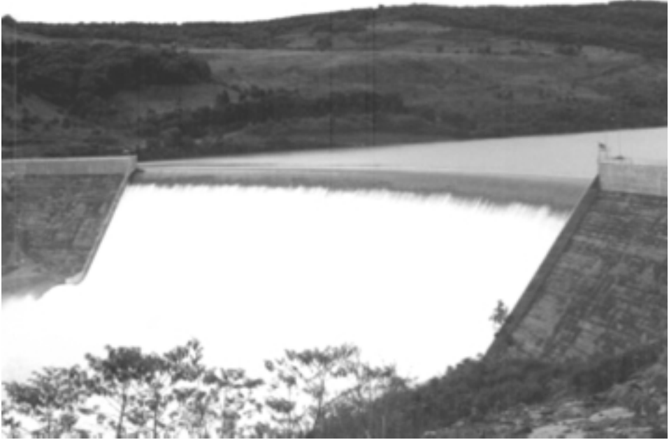
Fig. A-8.1 Photograph of Jordão dam with spillway in operation
