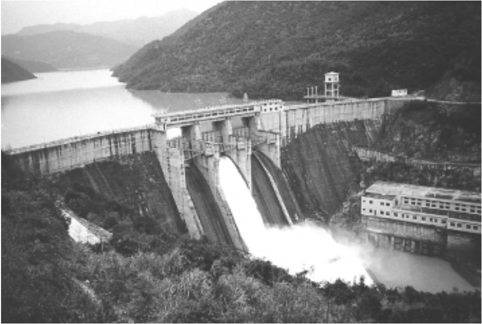
Fig. A-7.1 Photograph of Shanzai dam
