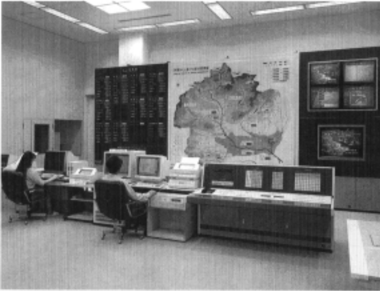
Fig. 5.40 Control room in the Tone River integrated dam office
